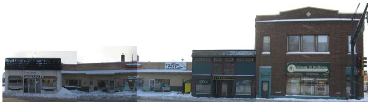
Existing building on Block 37 viewed from Highway 2.
