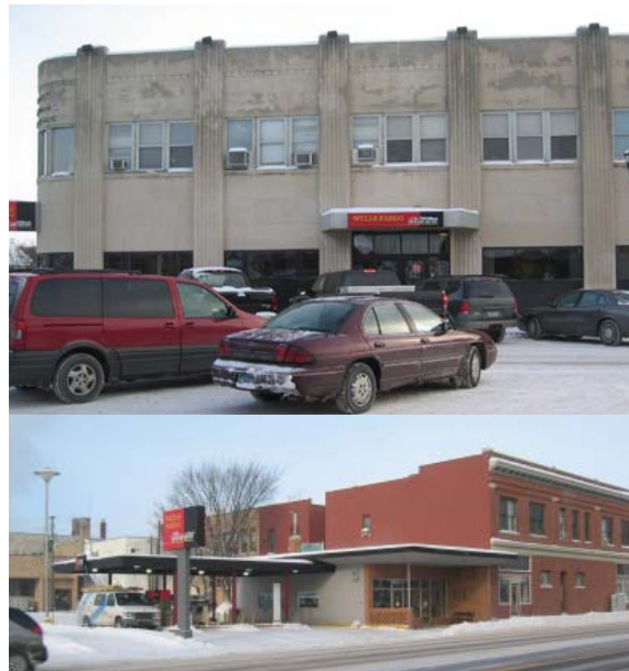
The relocation of Wells Fargo Bank and the related drive up banking facilities provides an important opportunity for redevelopment
