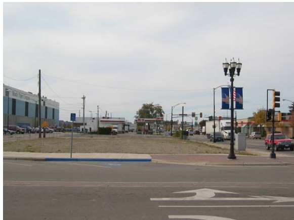
Vacant parcels and transportation (highway and rail) corridors impede the feeling that Downtown is a single and well connected district.
