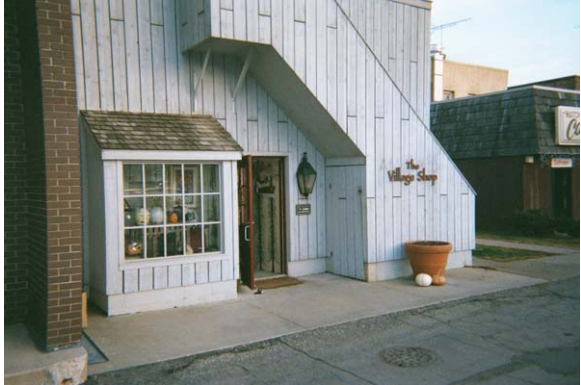
Rear building entrance in Hutchinson
