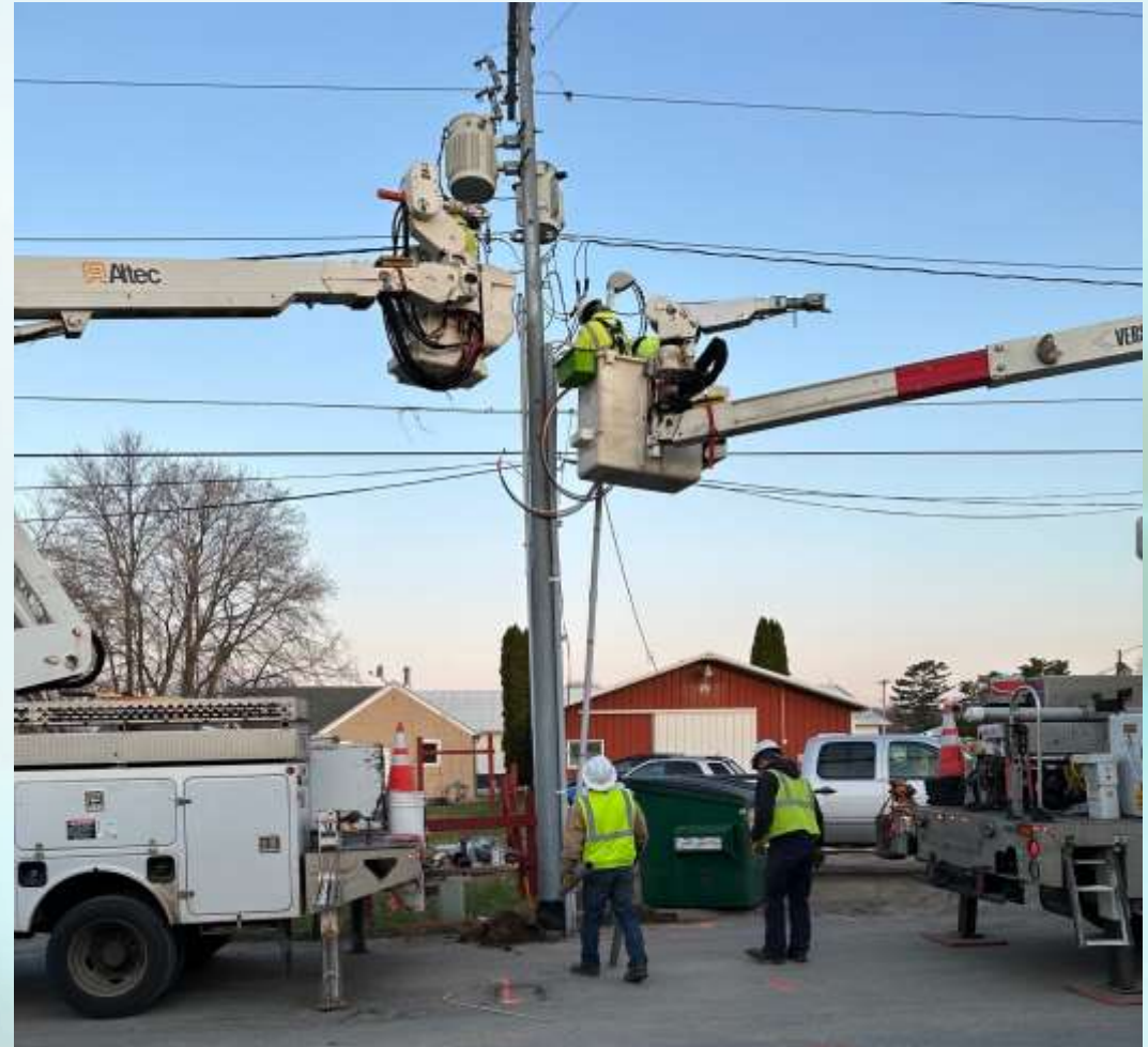
Early Morning Outage for Service Upgrade.
