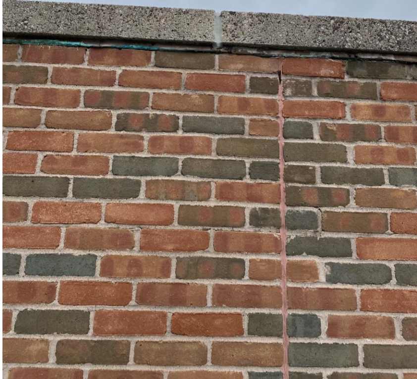
Photograph 26 – Sealant at masonry joints.
