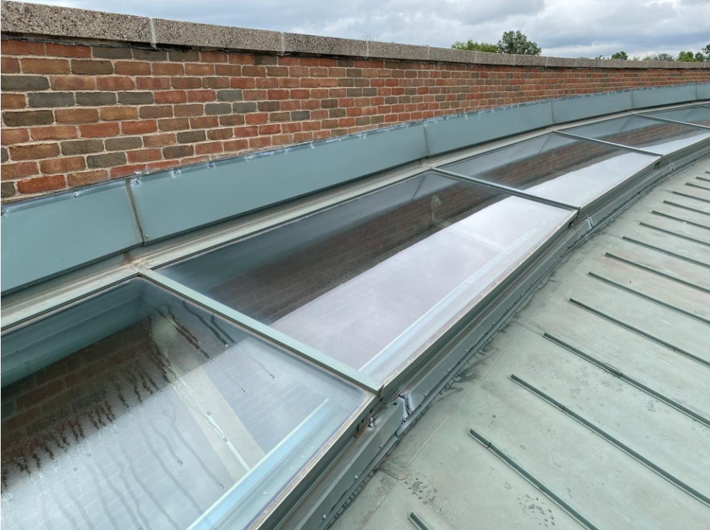
Photograph 19 – Skylight assembly at the roof.
