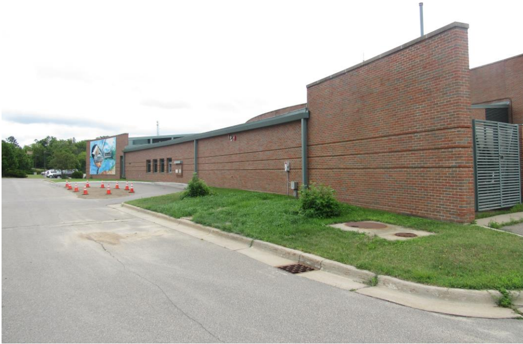
Photograph 3 – The north elevation of the library building.
