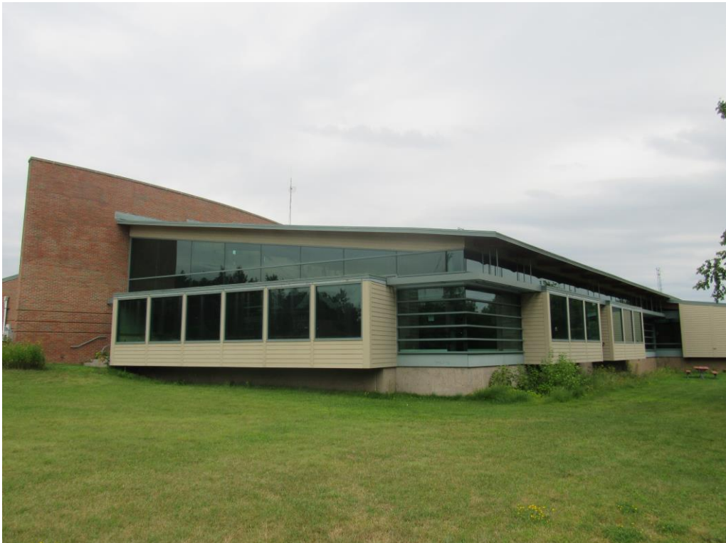
Photograph 2 – The west elevation of the library building.
