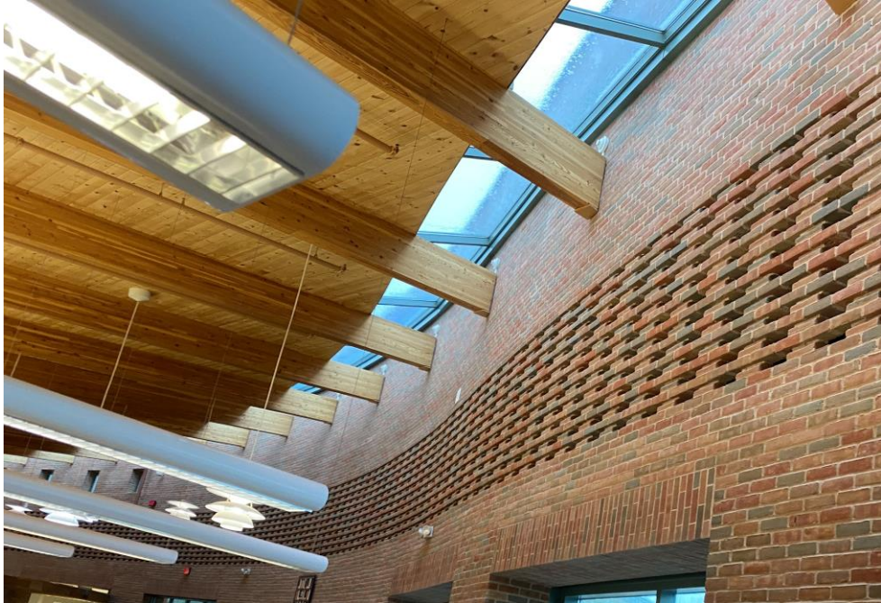
Photograph 20 – Interior view of skylight assemblies.
