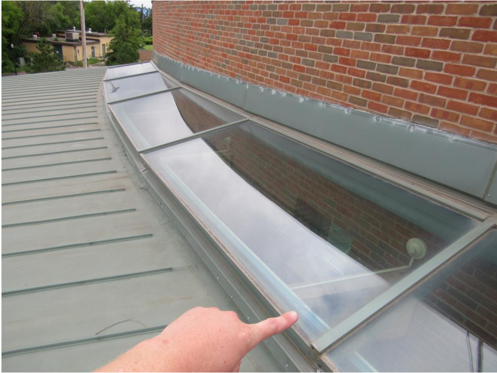
Photograph 10 – Water testing location at the skylights.
