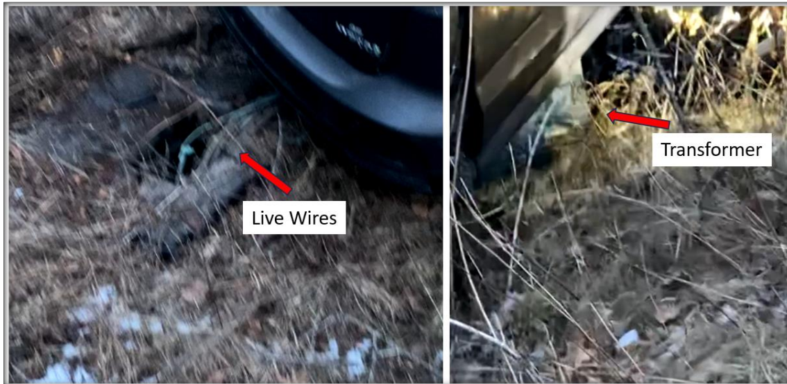
Figure 1: Vehicle Caused Outage
