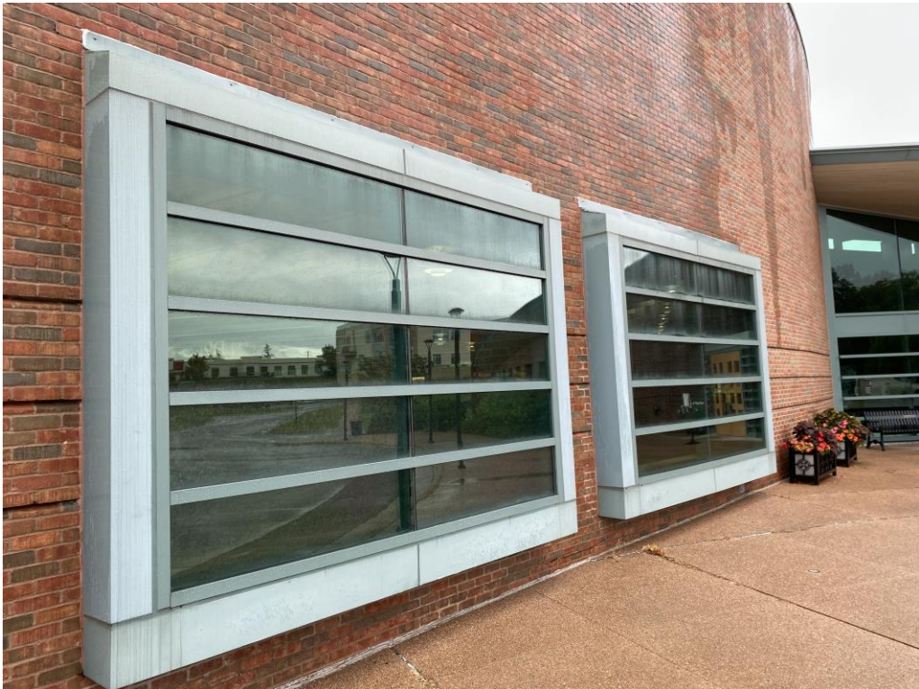
Photograph 4 – Bumpout window assembly near the main entrance.
