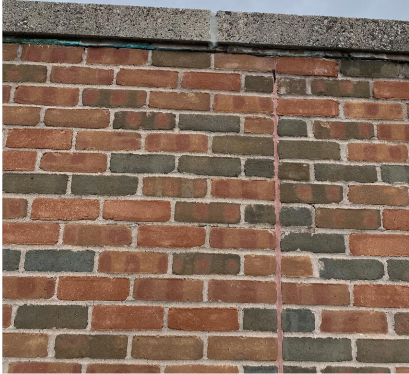
Photograph 26 – Sealant at masonry joints.
