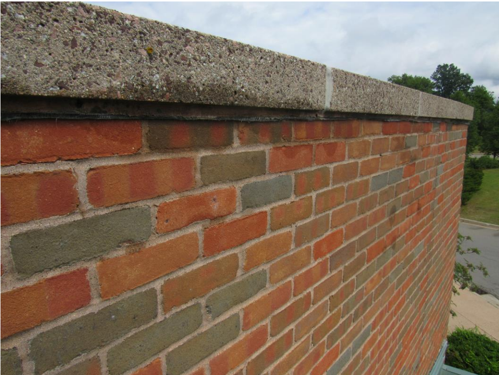
Photograph 15 – Wall cap details showing flashing conditions.
