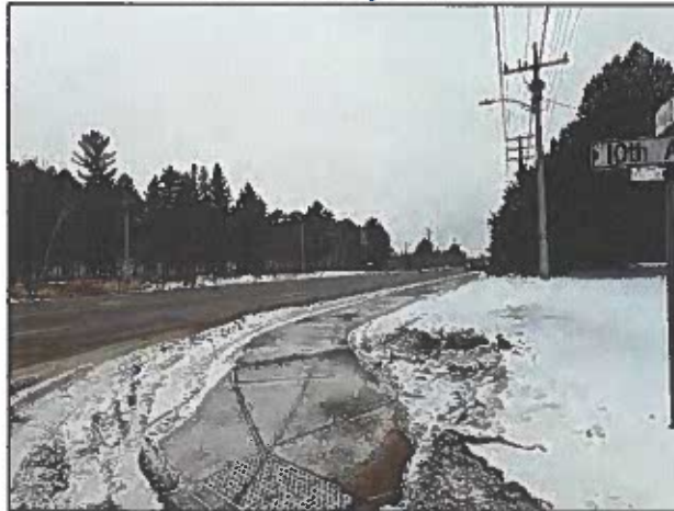
Looking west-northwesterly along U.S. Highway 2 E (TH 2) from NE 10 th Avenue
