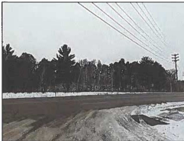
Looking southwesterly at the subject and area of the proposed acquisition from NE 1 st Street
