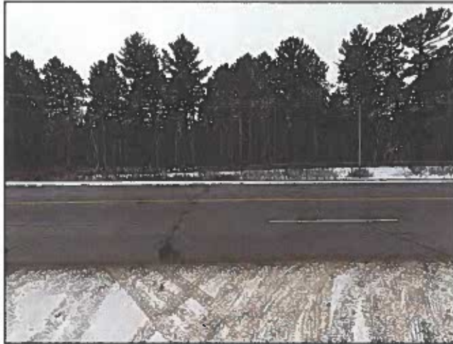
Looking southerly across U.S. Highway 2 E (TH 2) from NE 11 th Avenue. The subject and area of the proposed acquisition are to the right.
