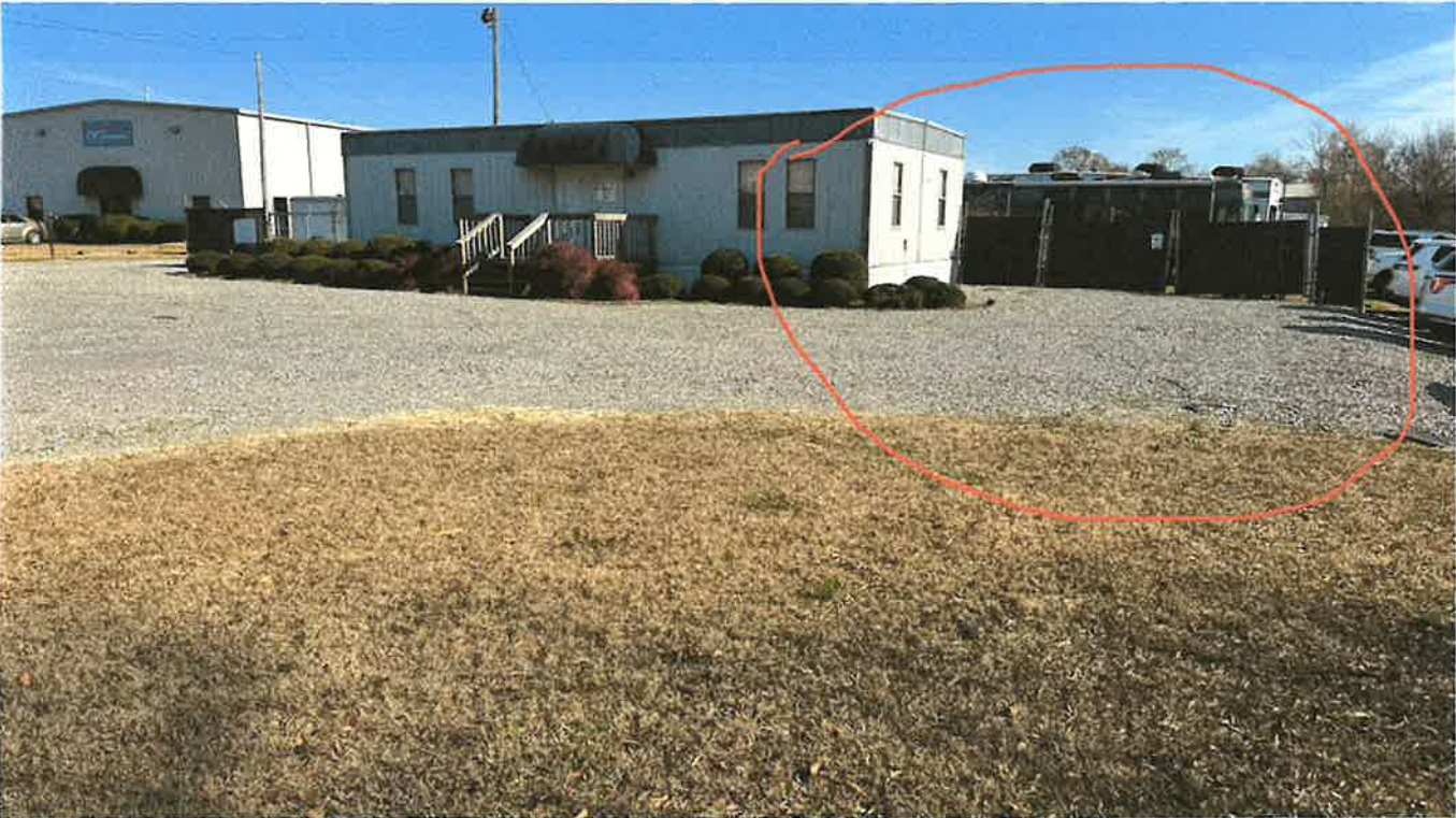
2. Good perspective of parking on the side of the office building.
