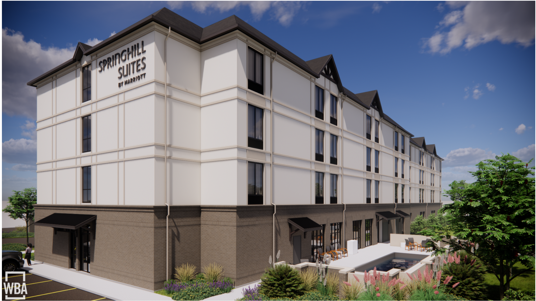
BACK VIEW (FROM NORTHEAST)
