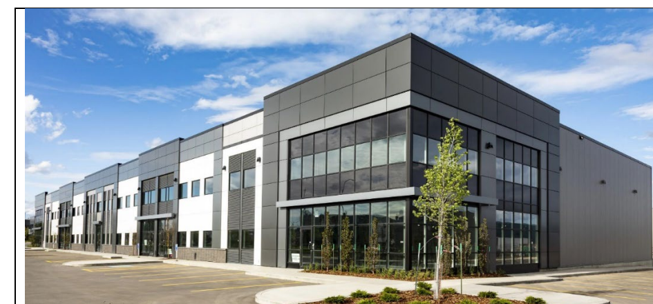
Figure 21. An industrial building articulated and given interest with fenestration, offsets in the facade and roof line, and color and material variation. Image from https://www.synergybuilds.com/featured-projects/mitchell-industrial-buildings
