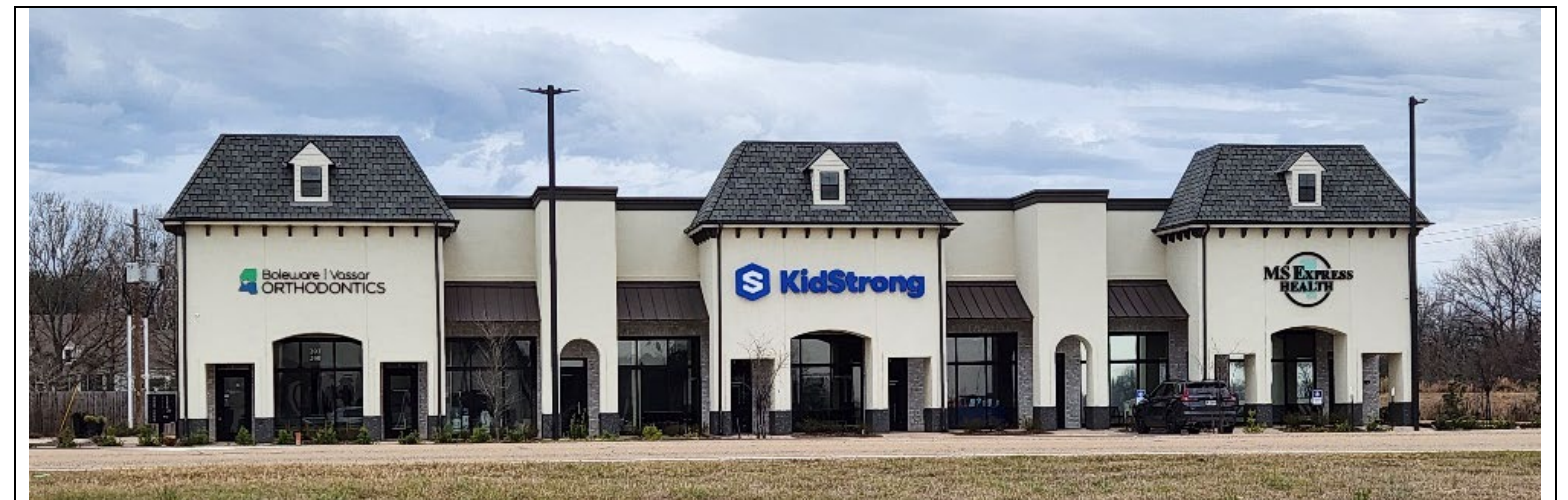
Figure 18. Differing shopfronts are uniquely distinguished by façade variations and details. The pictured building exhibits substantial articulation at each storefront.
