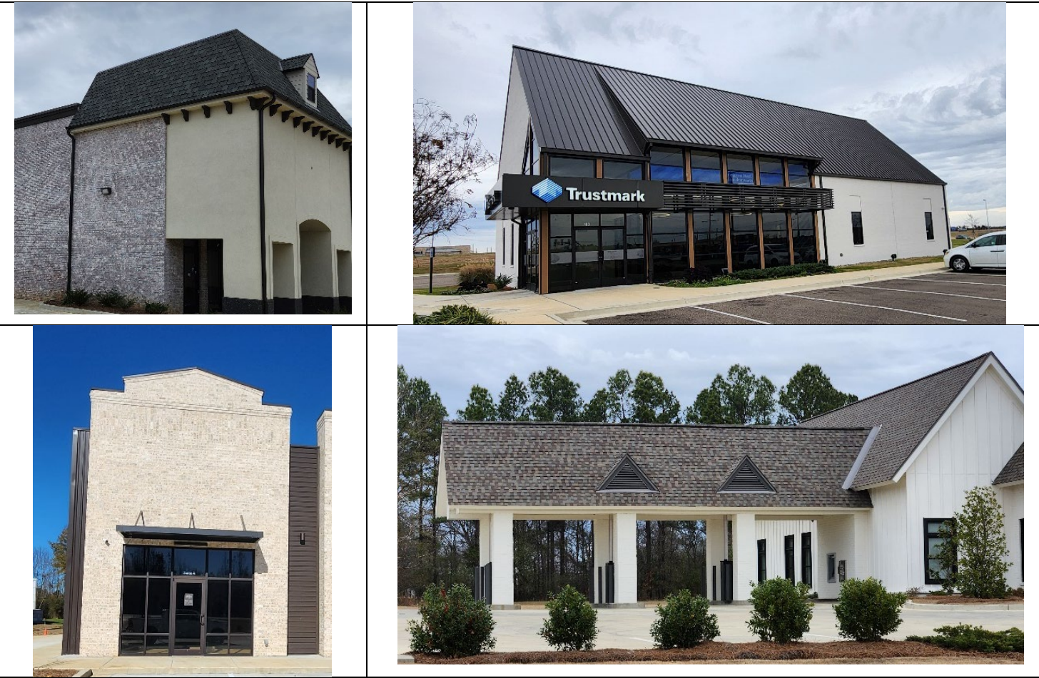
Figure 20. Top left, top right and lower left are acceptable roof configurations. Lower right: Drive through canopy and vertical supports design consistently with its parent building.
