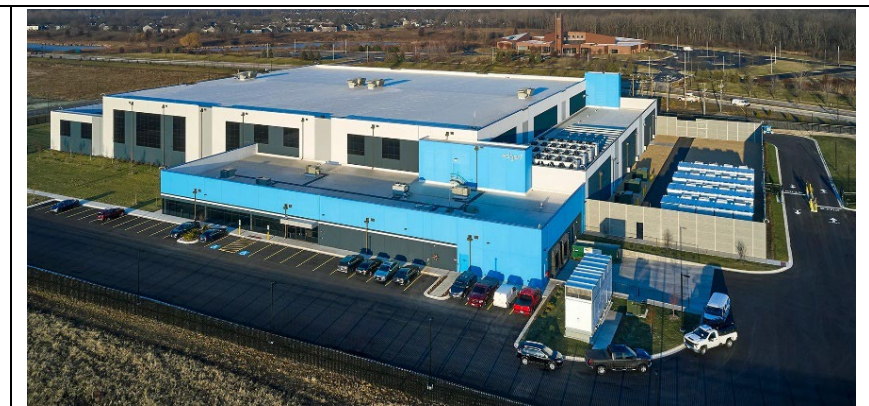
Figure 23. Step down, or single story portion of industrial building highlighted in blue, reduces the mass of the building. Image from https://www.naiop.org/research-and-publications/best-practices-in-data-center-development/
