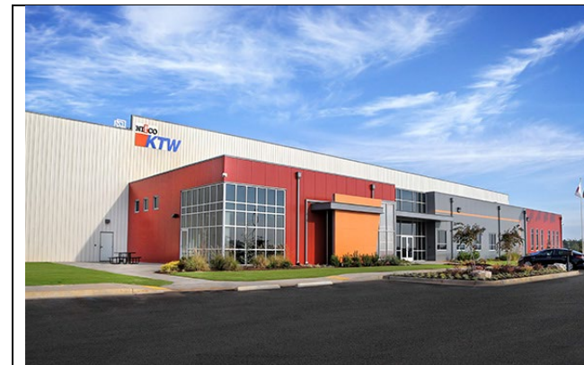
Figure 22. Distinct treatment of primary entrance and use of clerestory window. Image from https://www.nucorbuildingsgroup.com/industrial-manufacturing-building-solutions/
