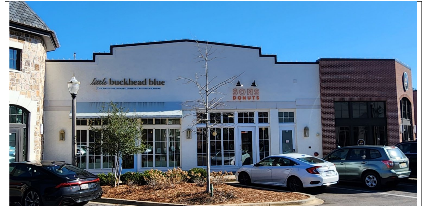
Figure 28. Example of a Village Mid Century building. Simple yet attractive design with large glazed frontage.
