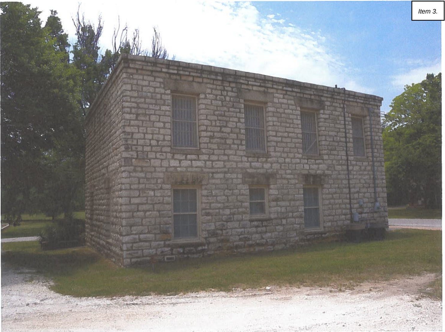
Glen Rose Historic Resource Survey, Site 52 (roll 6, exp. 7), Somervell County Jail, 106 Cedar Street, southwest to rear and southeast side.
