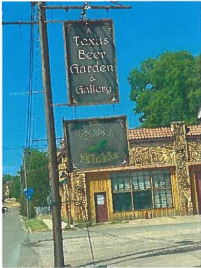
Old Sign. Replace with new metal sign. Logo cut out with green metal in between to make logo green
