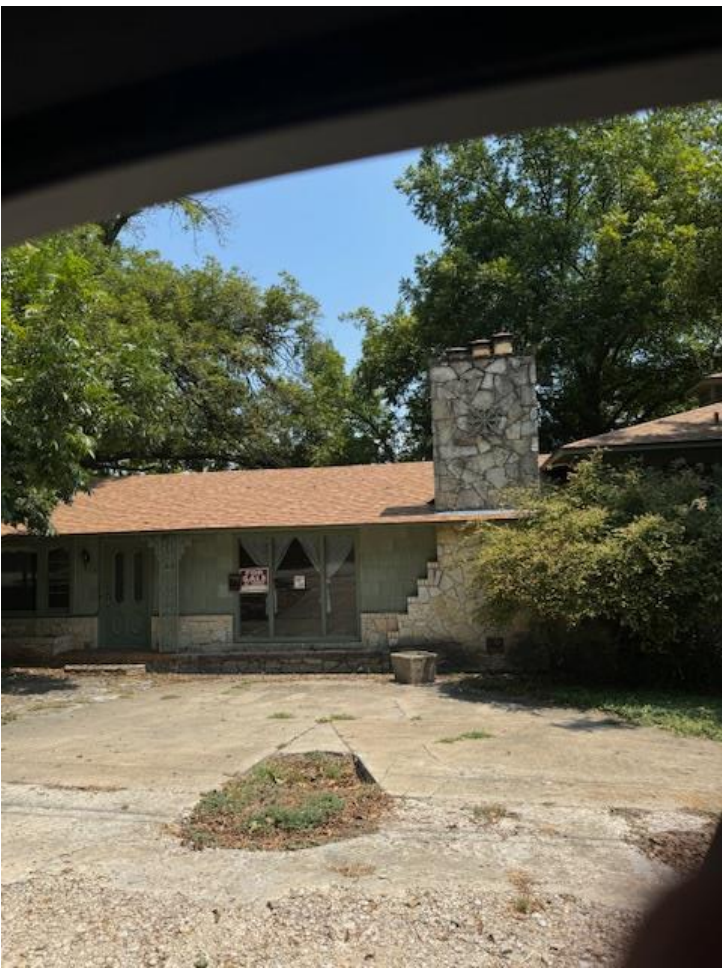
Recent photo with new roof.
