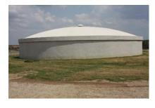
Project Description: Engineering design and construction administration for the Installation of 8 MGD pump station and 2.0 MG wire-wound, pre-stressed concrete ground storage tank.
