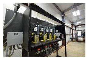
**Project Description:** Engineering design and construction administration for three reverse osmosis treatment plants for arsenic and fluoride removal (total Capacity of treatment 3.0 MGD)
