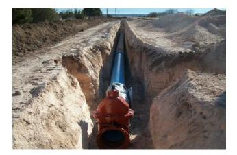
**Project Description**: Engineering design and construction administration for the Installation of a new raw water pump station and head tank located at Hords Creek Lake, approximately 44,000 LF of 16" raw water supply line and approximately 40,000 linear feet of water distribution lines.
