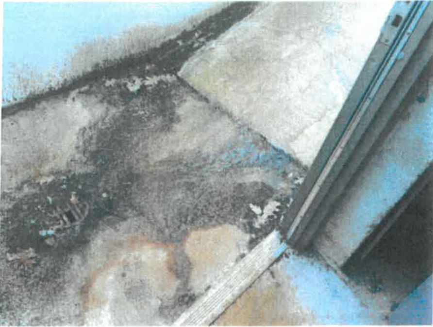
Photo 5: Exterior drain at landing of exterior walkway
