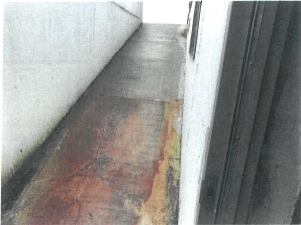
Photo 6: Exterior walkway from photo 5
