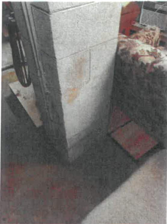
Photo 4: Patched masonry column (typ)
