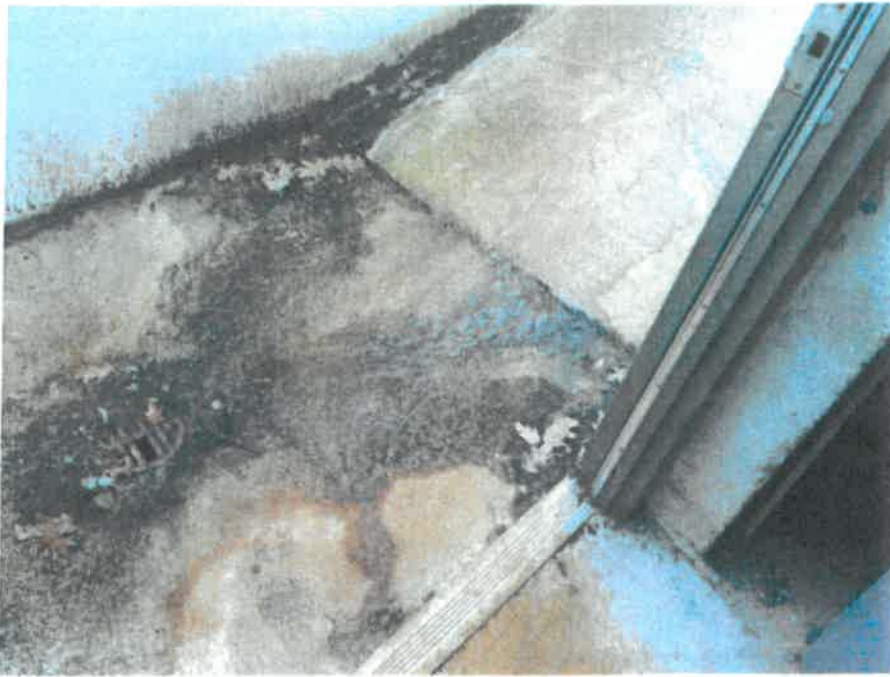
Photo 5: Exterior drain at landing of exterior walkway
