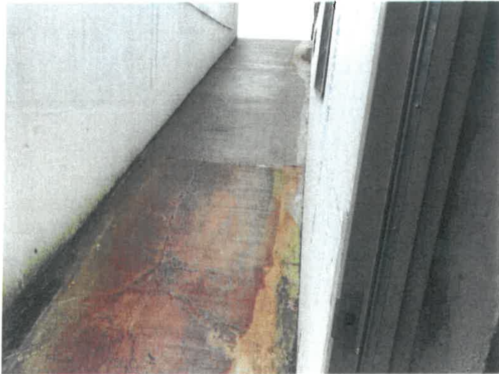
Photo 6: Exterior walkway from photo 5
