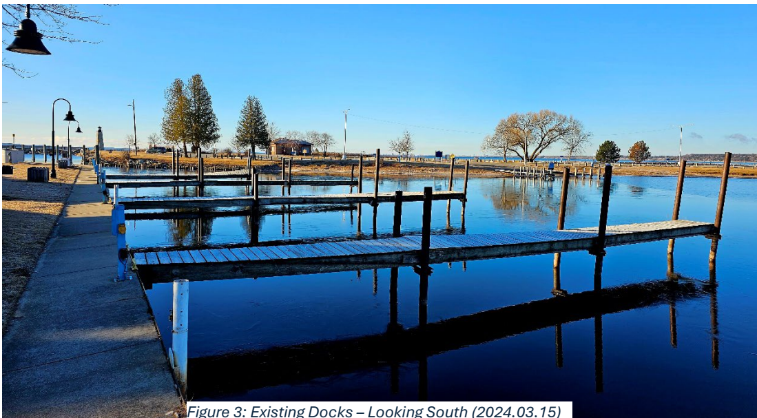
Figure 3: Existing Docks – Looking South (2024.03.15)
