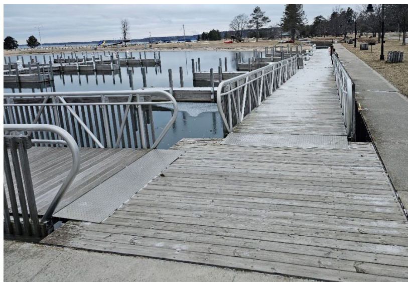
Figure 2: Phase I Flotation Docking – Northeast Looking South (2024.03.18)
