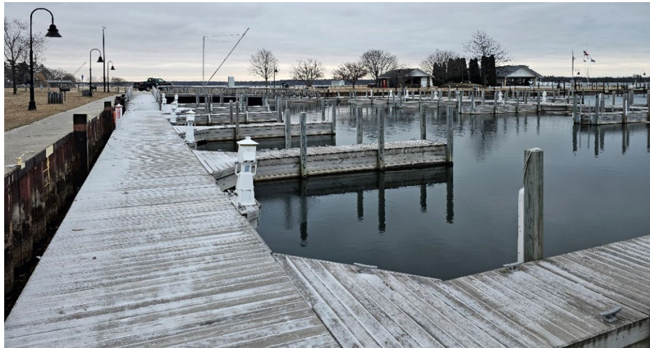
Figure 1: Phase I Flotation Docking – West End of Docks – Looking Southeast (2024.03.18)
