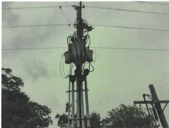
POLE-MOUNTED TRANSFORMERS
