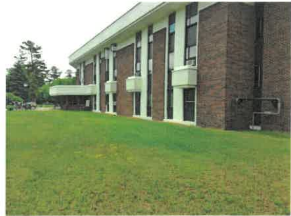
NORTHEAST ELEVATION OF SUBJECT BUILDING
