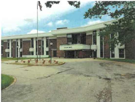
WEST ELEVATION OF SUBJECT BUILDING
