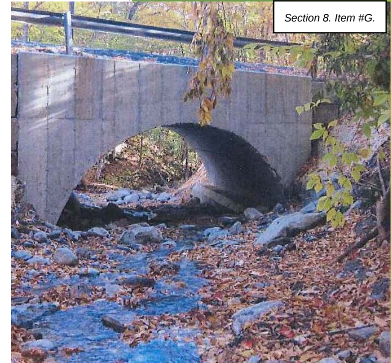
New bridge, Duxbury
