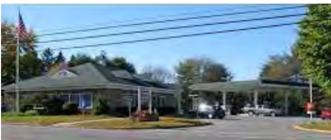
Figure 3.1 - Fuel pumps in rear of building.
