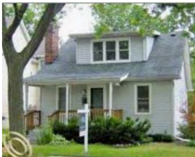
Figure 10.2 - Shed dormer, with a single, inclined roof.
