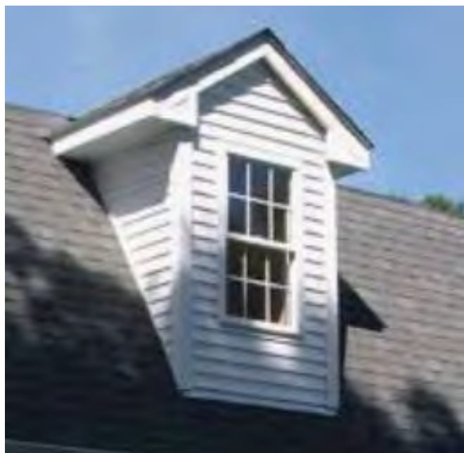
Figure 10.1 - Dog house dormer, with gable roof
