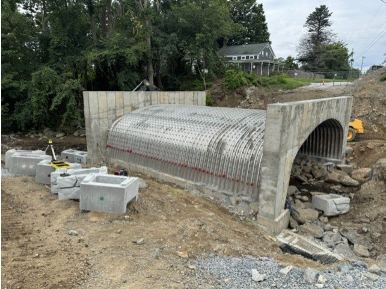
Bridge construction: arch installation and site preparation
