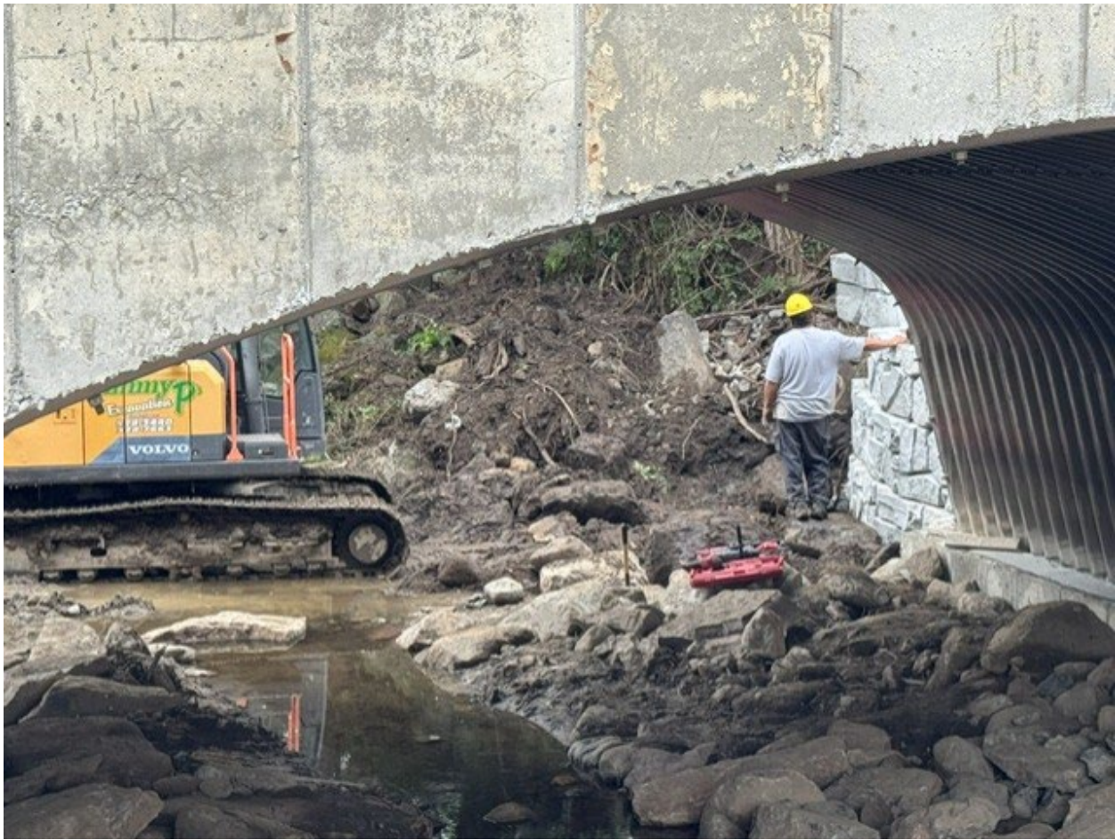
Bridge construction progress during the reporting period
