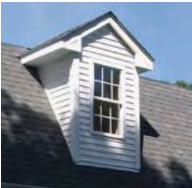
Figure 10.1 - Dog house dormer, with gable roof
