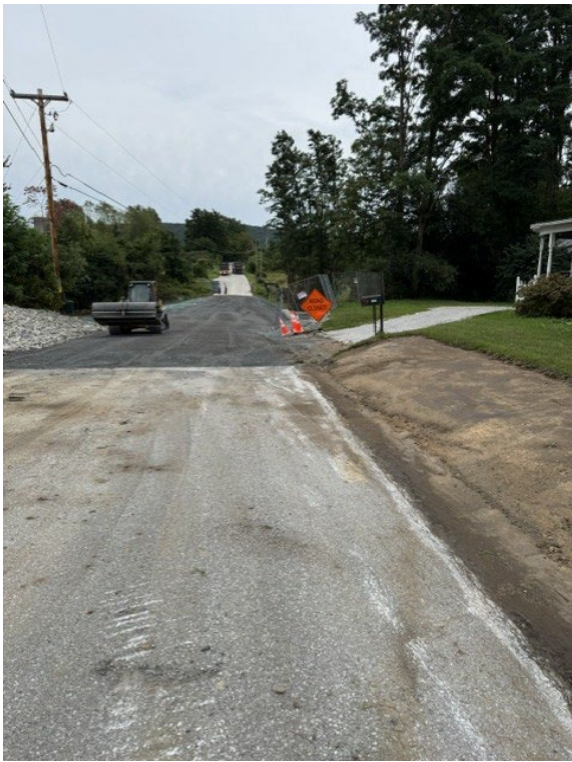
Bridge finished waiting on paving
