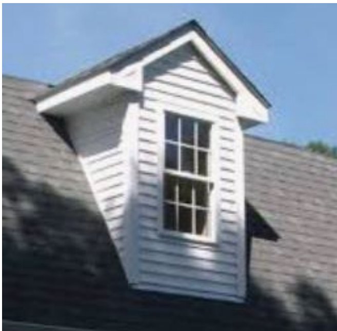
Figure 10.1 - Dog house dormer, with gable roof
