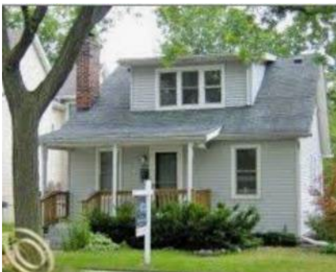
Figure 10.2 - Shed dormer, with a single, inclined roof.
