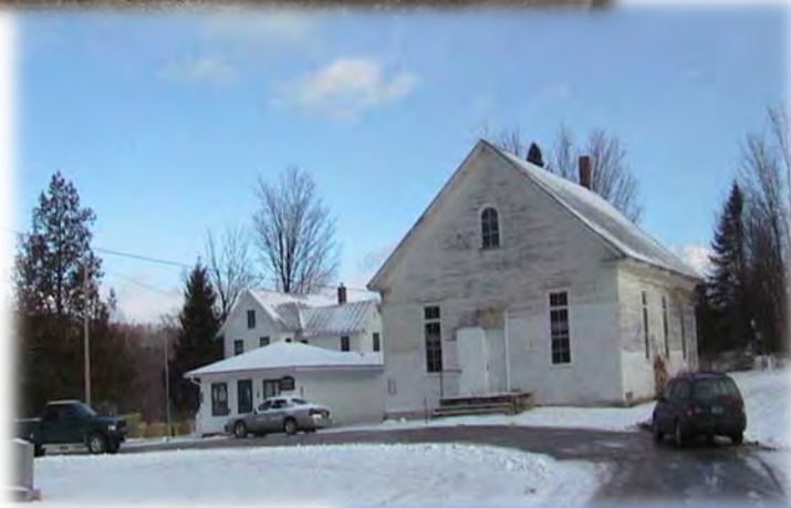
Berkshire Town Hall Before Renovations (Photo credit: NRPC)
