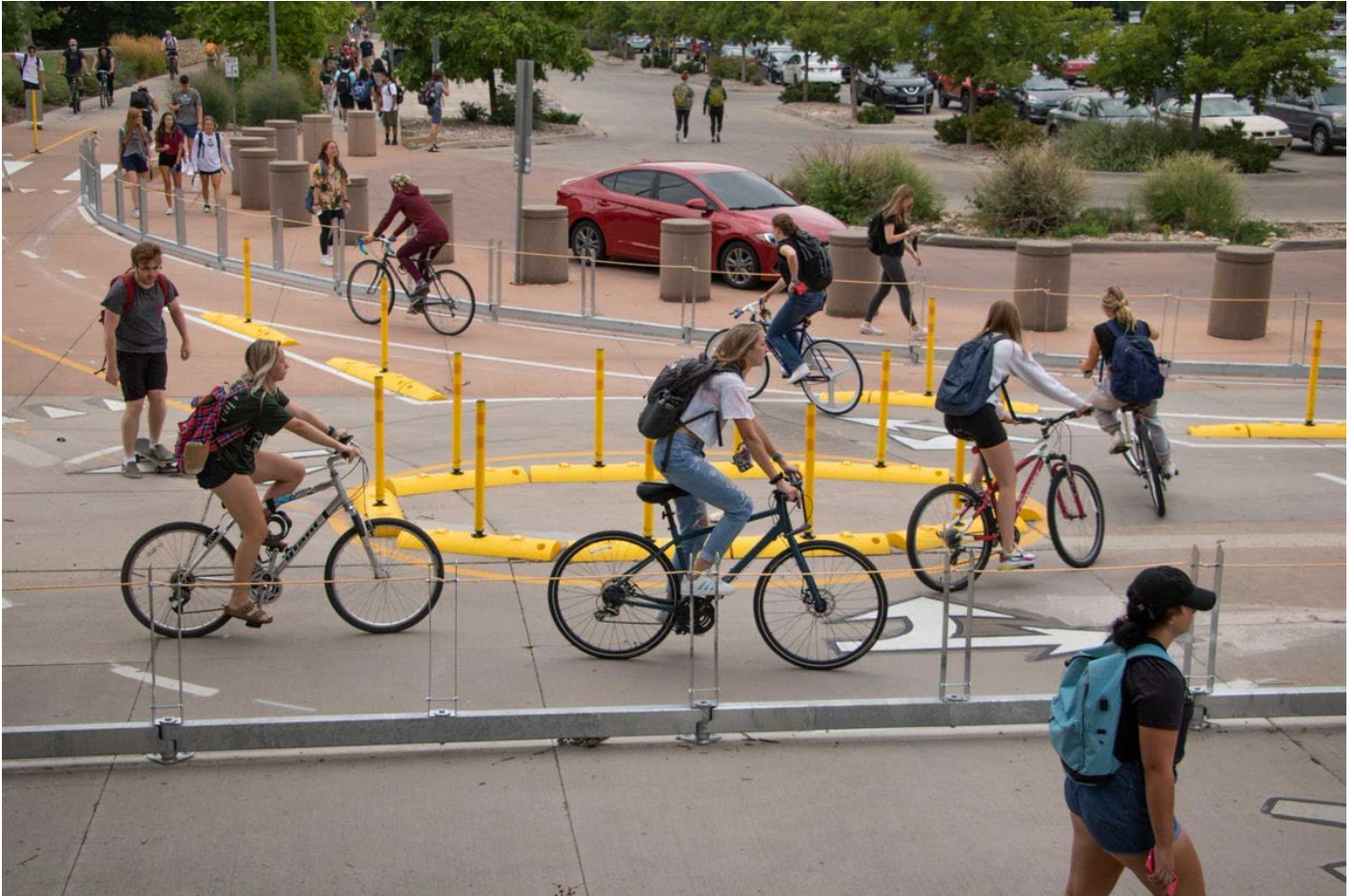
A bicycle roundabout created at CSU with rubber curbing and flexible bollards is an example of an innovative treatment using low-cost materials that are easily adjusted. Source: CSU.
