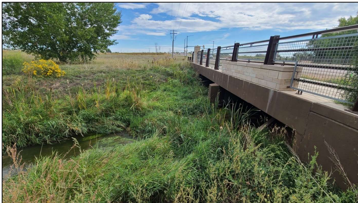
Photo 2. Prospect Corridor Improvements: Facing east, north side of Boxelder Creek and riparian corridor. Site was heavily vegetated which continued on the south side of the Prospect Road bridge.
