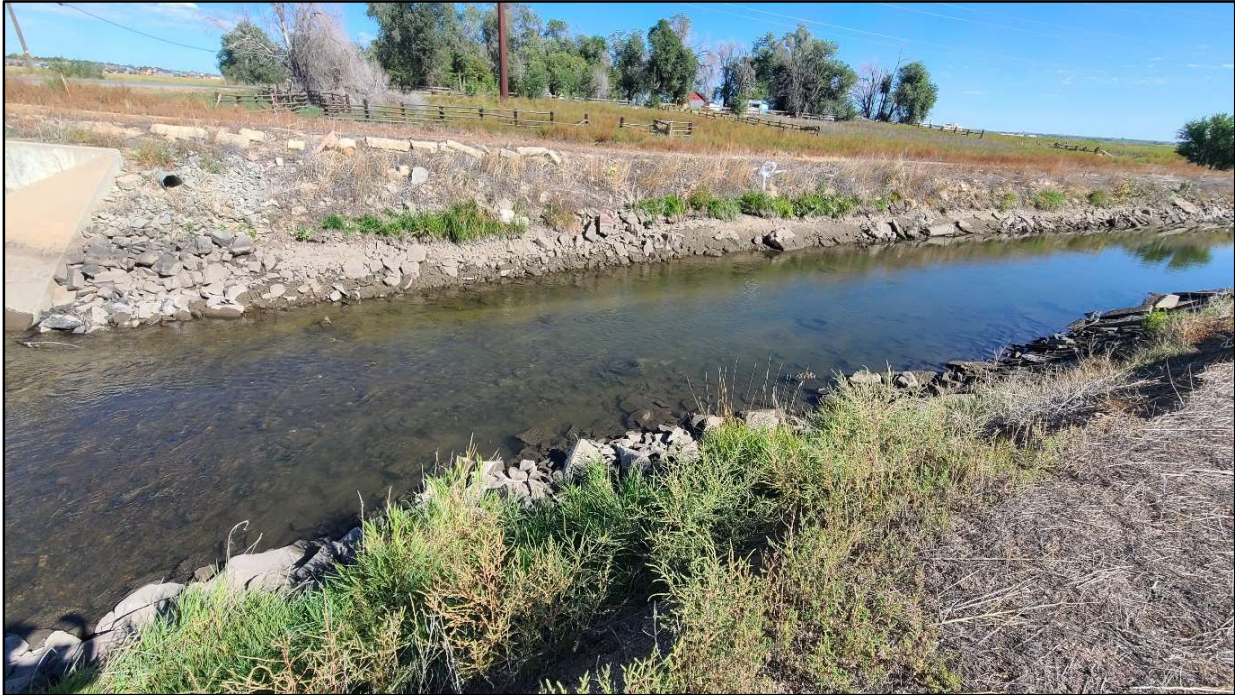
Photo 12. Timberline Road North – Segment 2: East side of Timberline Road (Segment 2) at the crossing of the Larimer and Weld Canal. Canal had steep banks and was armored with riprap. Vegetation was relatively sparse.
