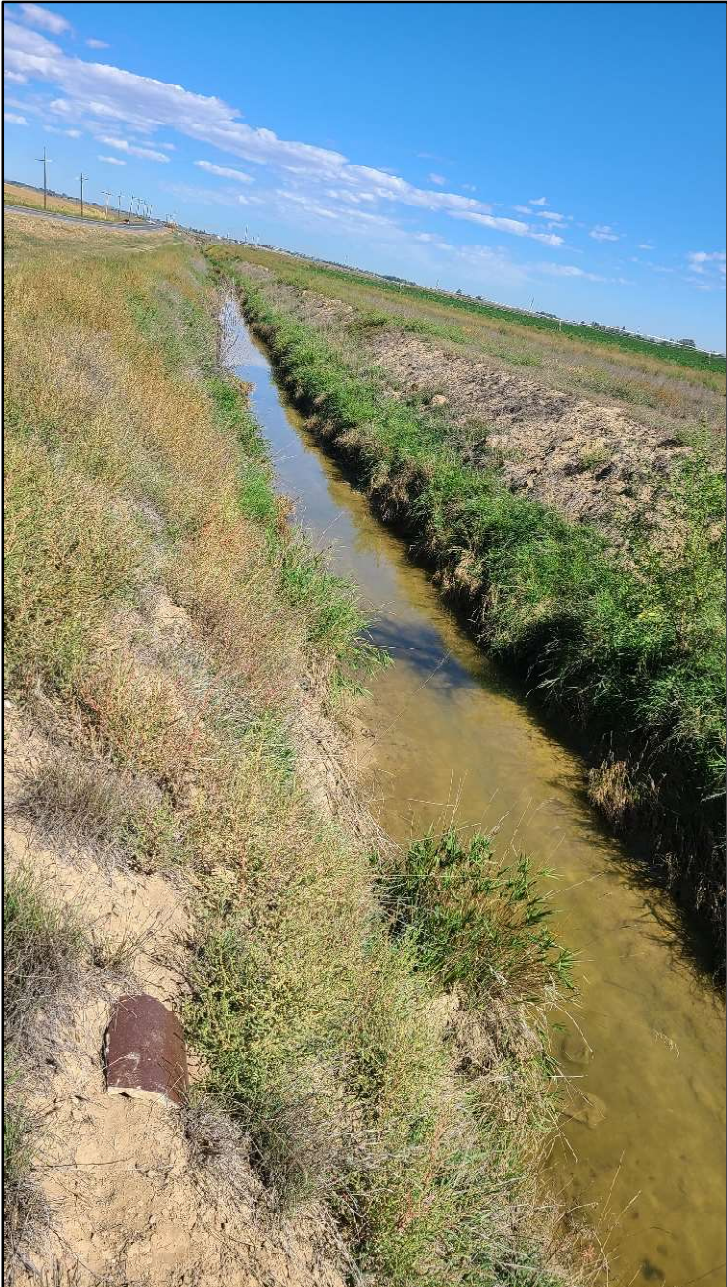
Photo 13. Timberline Road North – Segment 2: Facing north, the Number 8 Canal, parallel to Timberline Road (segment 2). Channel had steep vegetated banks which were eroding in areas. The canal continues south where it eventually drains into the Larimer and Weld Canal.
