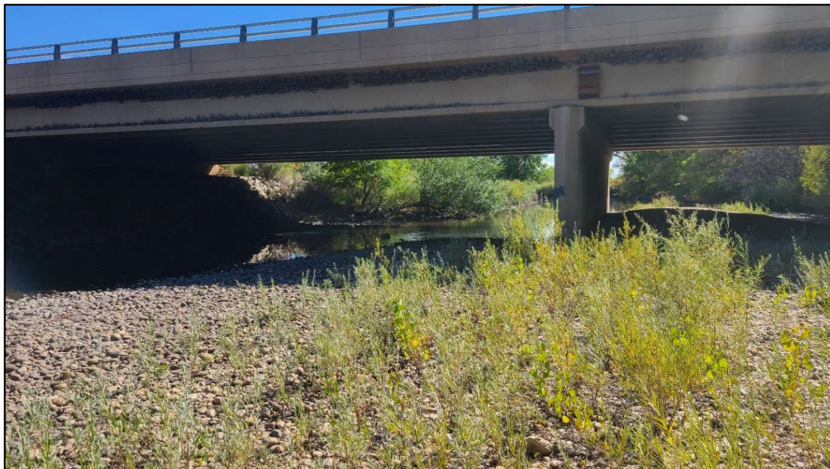
Photo 1. Prospect Corridor Improvements: Facing south, Cache la Poudre River flowing beneath Prospect Road bridge. Evidence of bird and bat habitat was seen on the bridge. East riparian corridor was steep and heavily vegetated.
