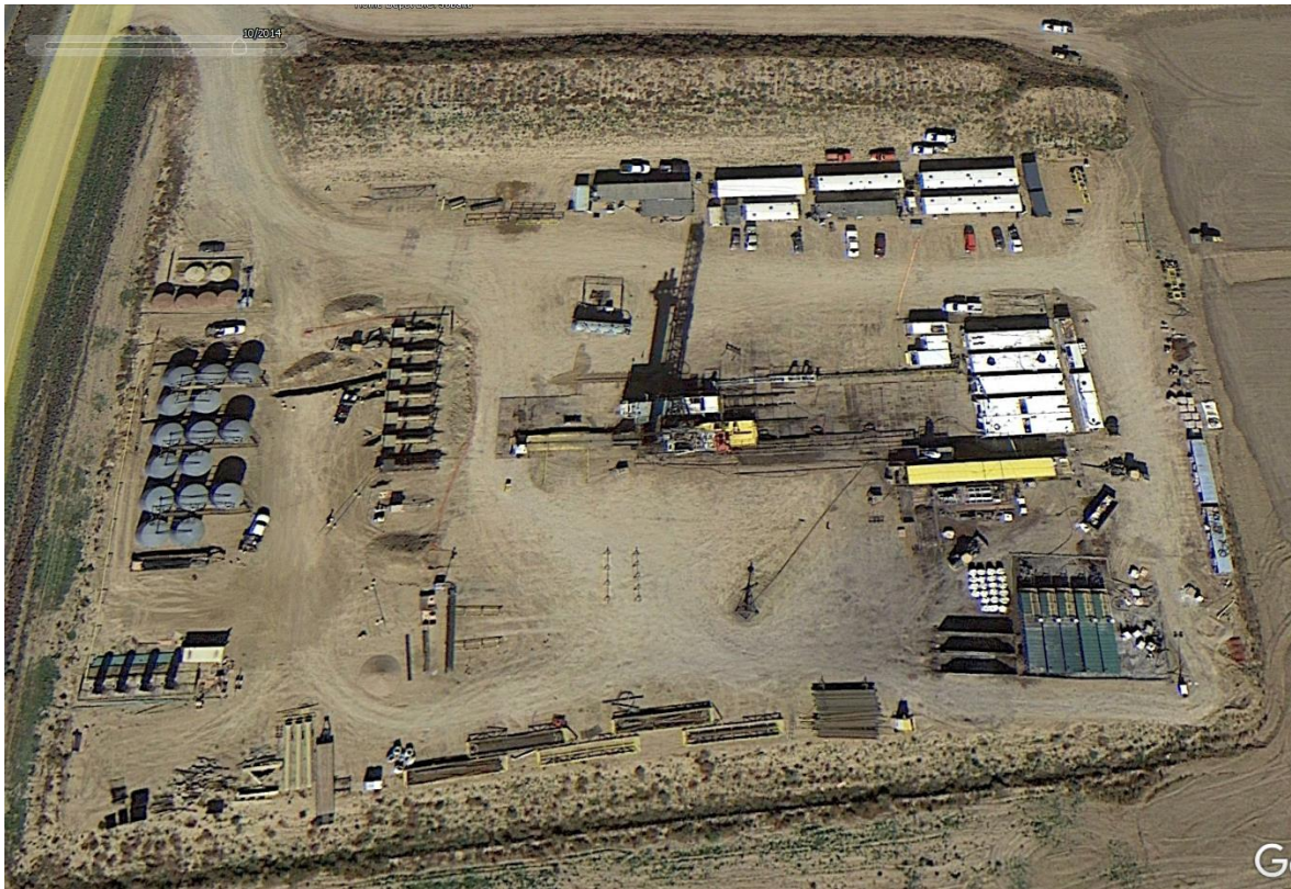
Figure 6: A pre-production 15-acre site drilling multiple long horizontal wells showing the drill rig and associated equipment.
