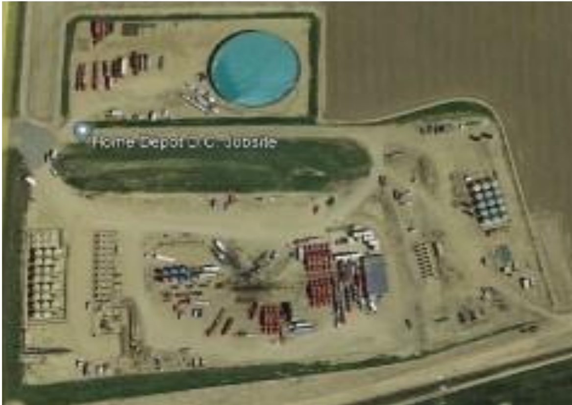
Figure 7: A pre-production 15-acre site drilling multiple long horizontal wells during hydraulic fracturing of the long horizontal wells.
