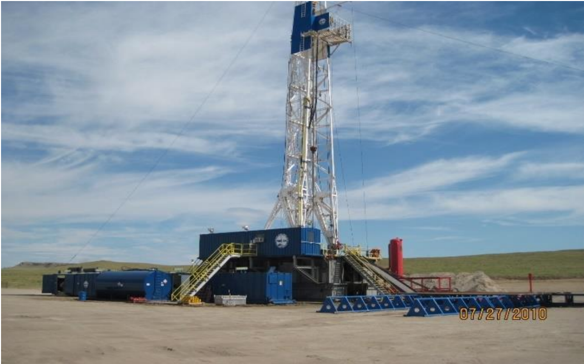
Figure 4: A typical drill rig use to drill a deep vertical hole.
