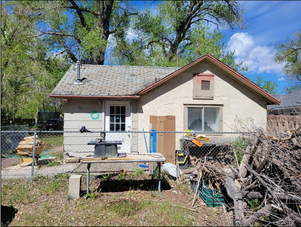
Figure 8: 724 Martinez, east elevation, view west (Image #101921, R. Shields, 5/14/2024).
