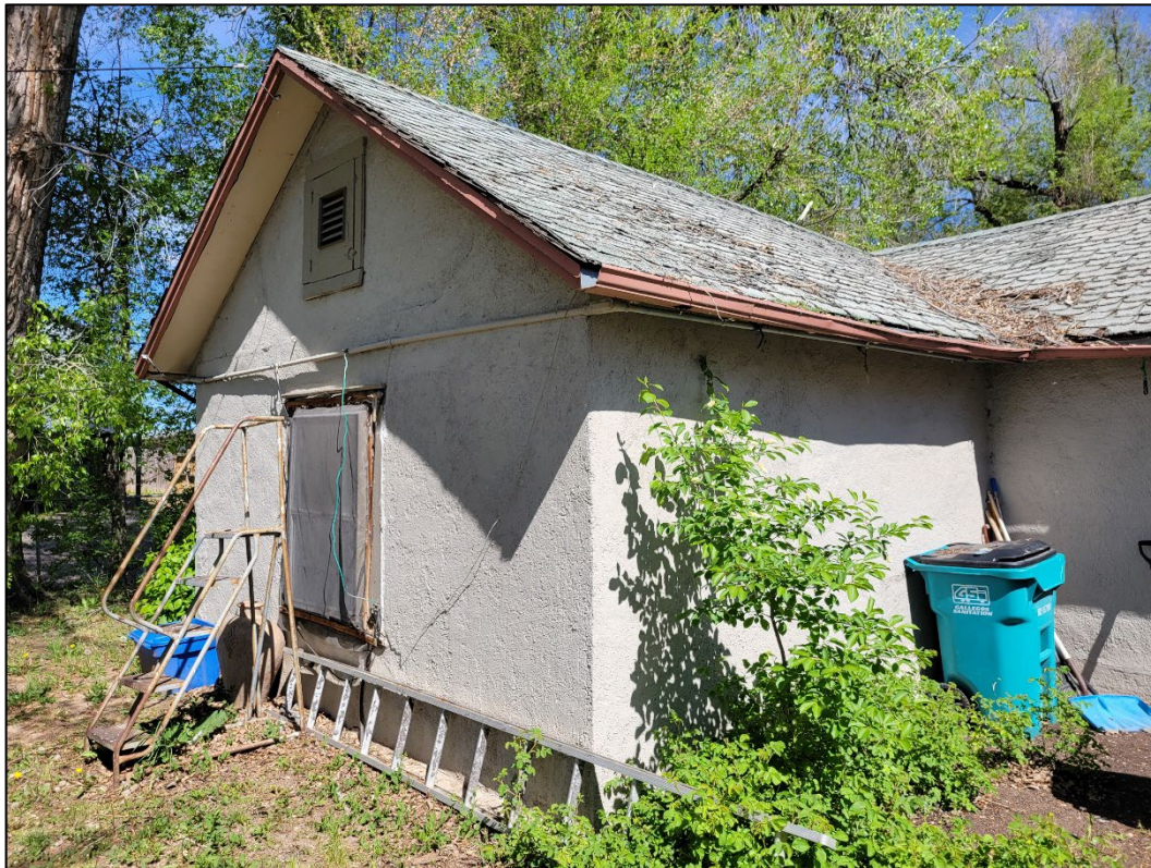
Figure 12: 724 Martinez, west end of south elevation, view northwest (Image #101251, R. Shields, 5/14/2024).
