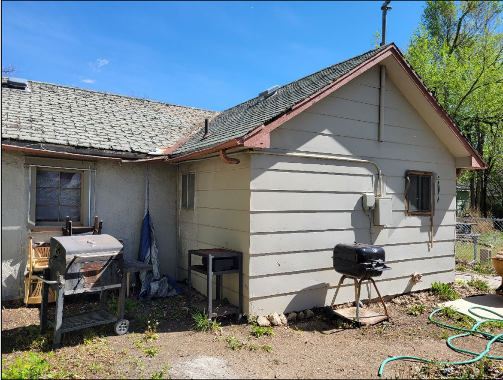
Figure 10: 724 Martinez, east end of south elevation, view northeast (Image #101230, R. Schields, 5/14/2024).
