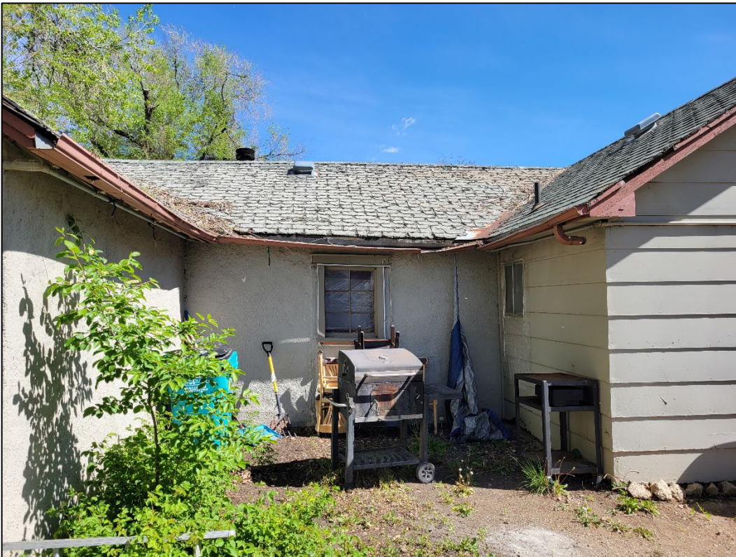
Figure 11: 724 Martinez, central portion of south elevation, view north (Image #101234, R. Schields. 5/14/2024).
