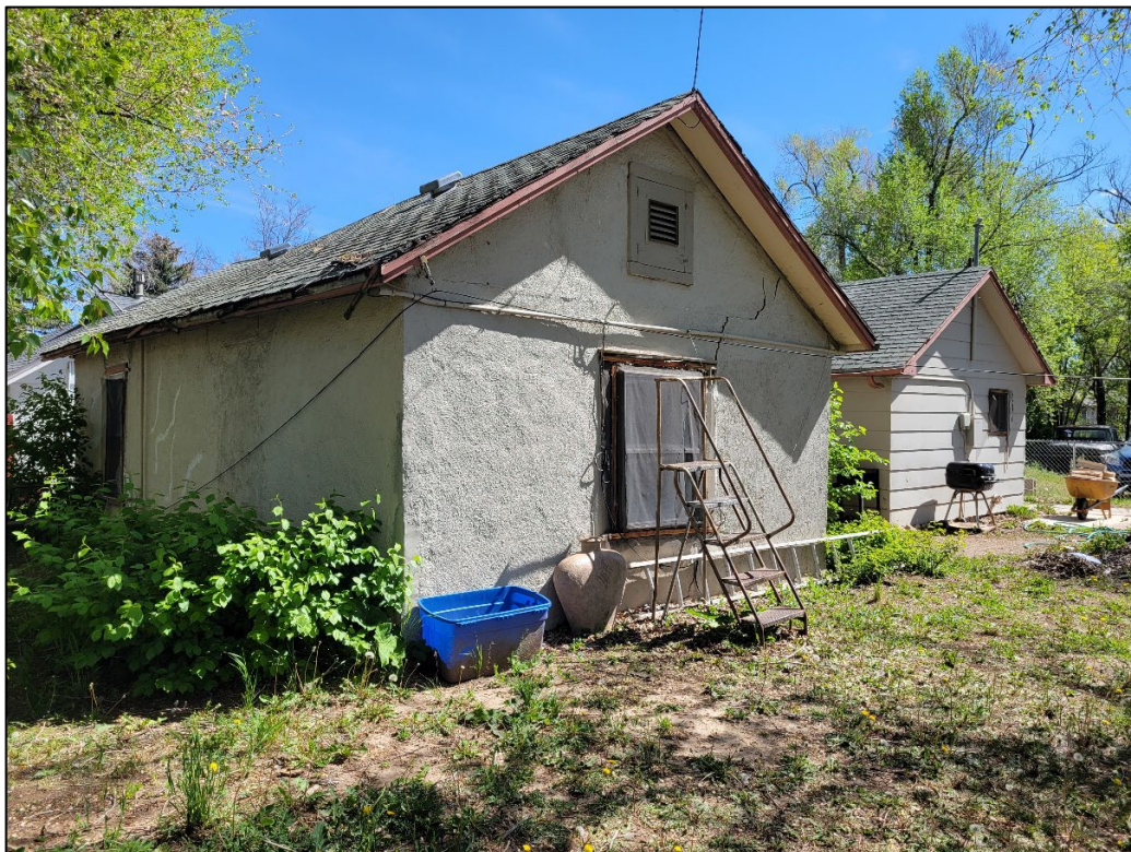
Figure 13: 724 Martinez, west and south elevations, view northeast (Image #101315, R. Shields, 5/14/2024).
