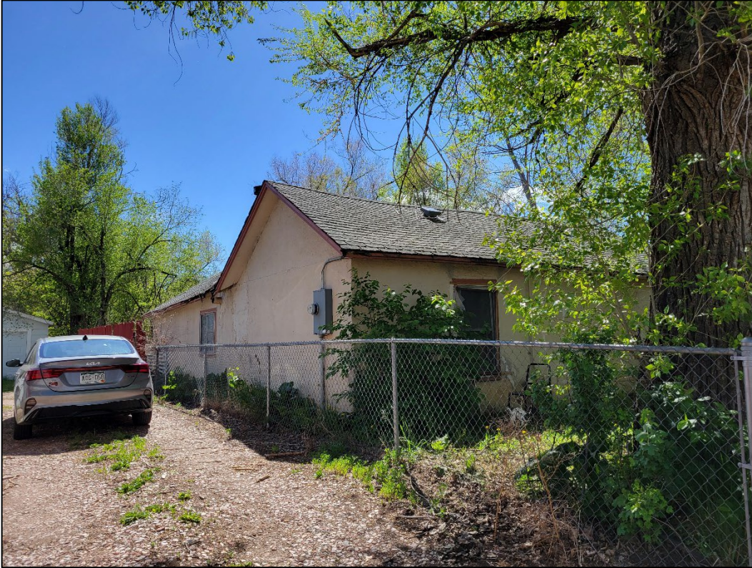
Figure 14: 724 Martinez, north and west elevations, view southeast (Image #102135, R. Shields, 5/14/2024).
