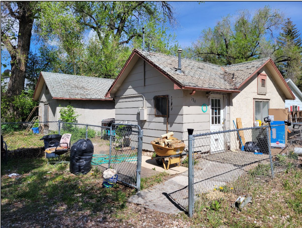
Figure 9: 724 Martinez, south and east elevations, view northwest (Image #101907, R. Shields, 5/14/2024).
