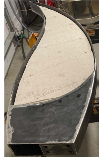
Cement board screwed to steel support bars.
