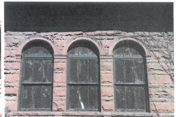
REMOVE PLYWOOD FROM WINDOWS (SHOWN COMPLETED) RENOVATE WINDOWS WITH NEW INSULATED GLAZING REFURBISH WINDOW FRAMES
