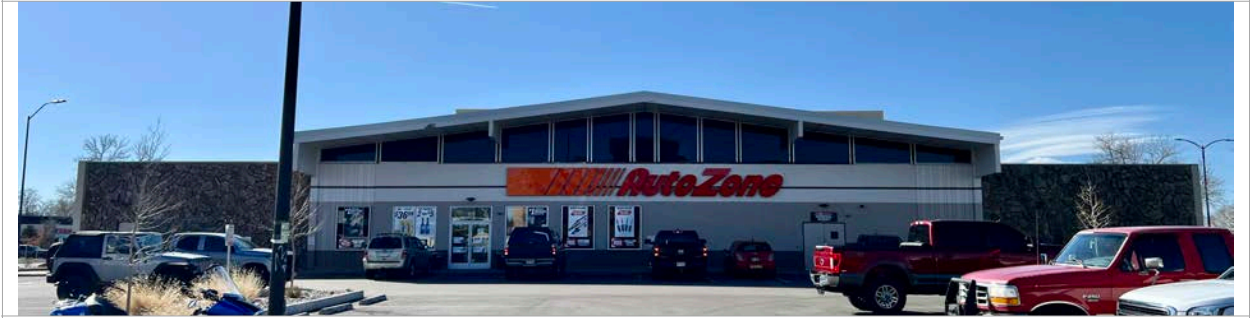
76. Auto Zone, 105 West Prospect Rd. Unknown construction date, not eligible for landmarking per the City of Fort Collins Historic Resources Planning Map. Note despite having many similar features to the dealership at 2601 South College Ave., such as CMU construction, stone veneer siding, a large gable roof, exposed rafters, and large amounts of glass, this building is not eligible for landmarking. Image courtesy of BEE. 2024.
