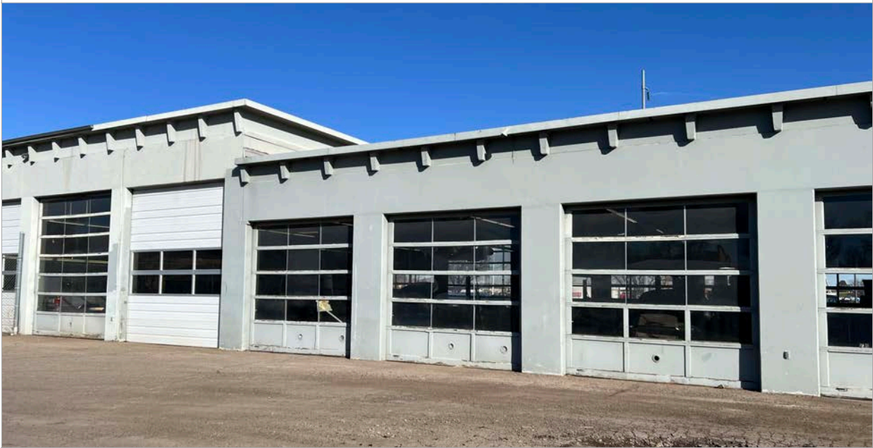
33. South Elevation - Service center, bays 5-11. Note more of the original garage doors on this elevation. Image courtesy of BEE. 2024.
