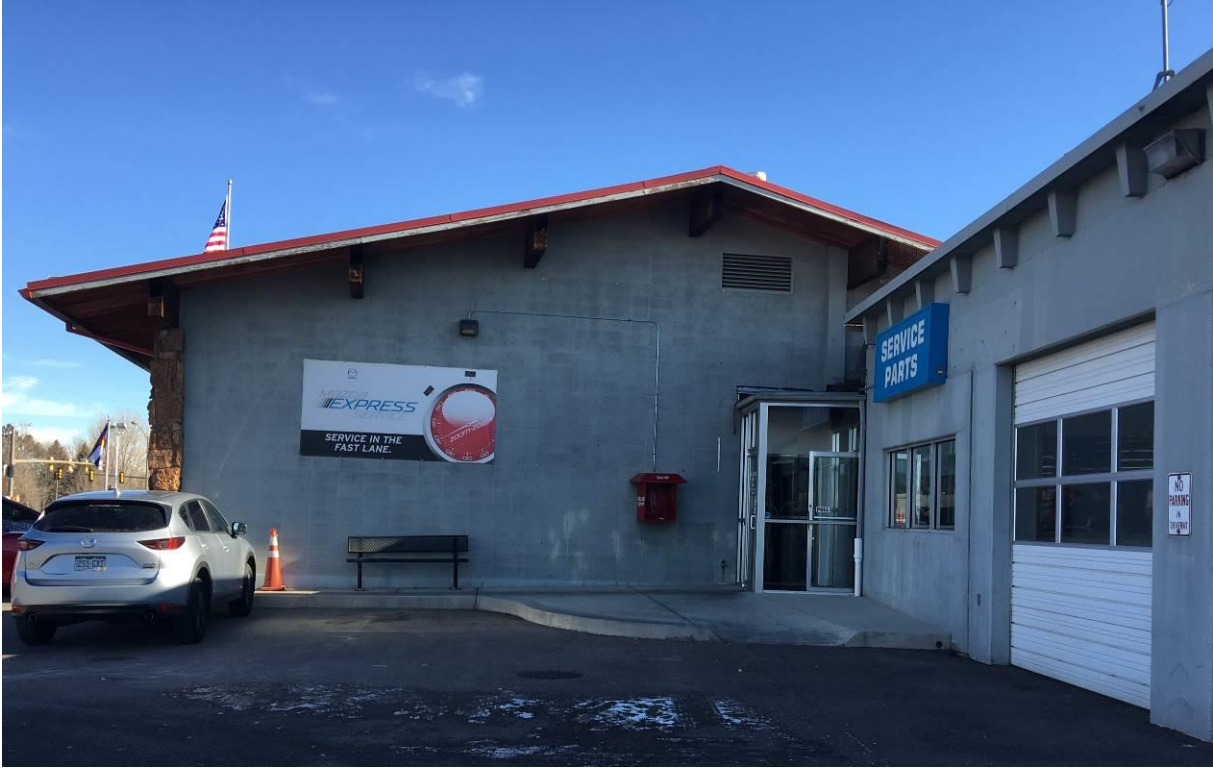
5LR.14283 – Spradley-Barr Parts and Service Entry (Foyer) (Bldg. A) Western elevation. Northern elevation of the Service Bay Section. Looking east. December 2017. Image 5LR.14283g.
