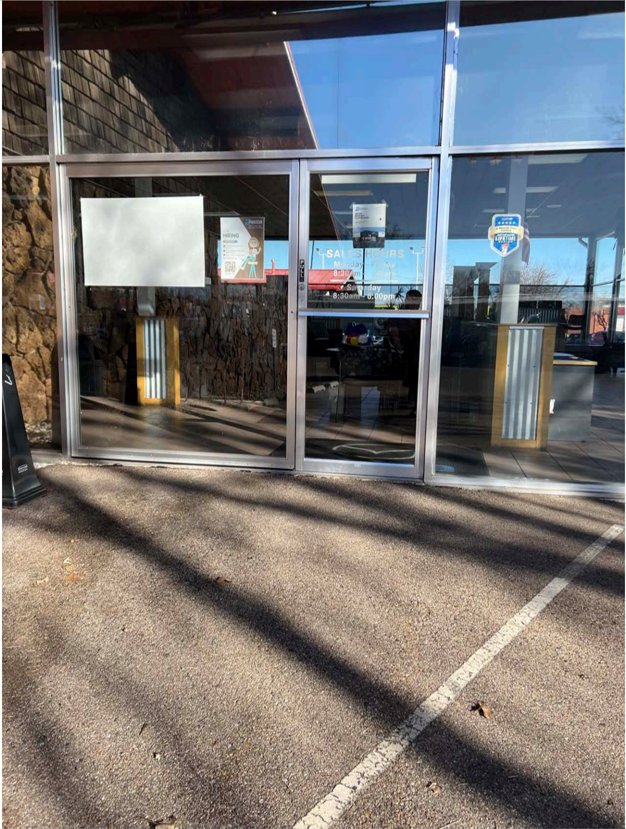
42. South Elevation - Detail of the door and hinged window that open to allow cars into the showroom. Image courtesy of BEE. 2024.
