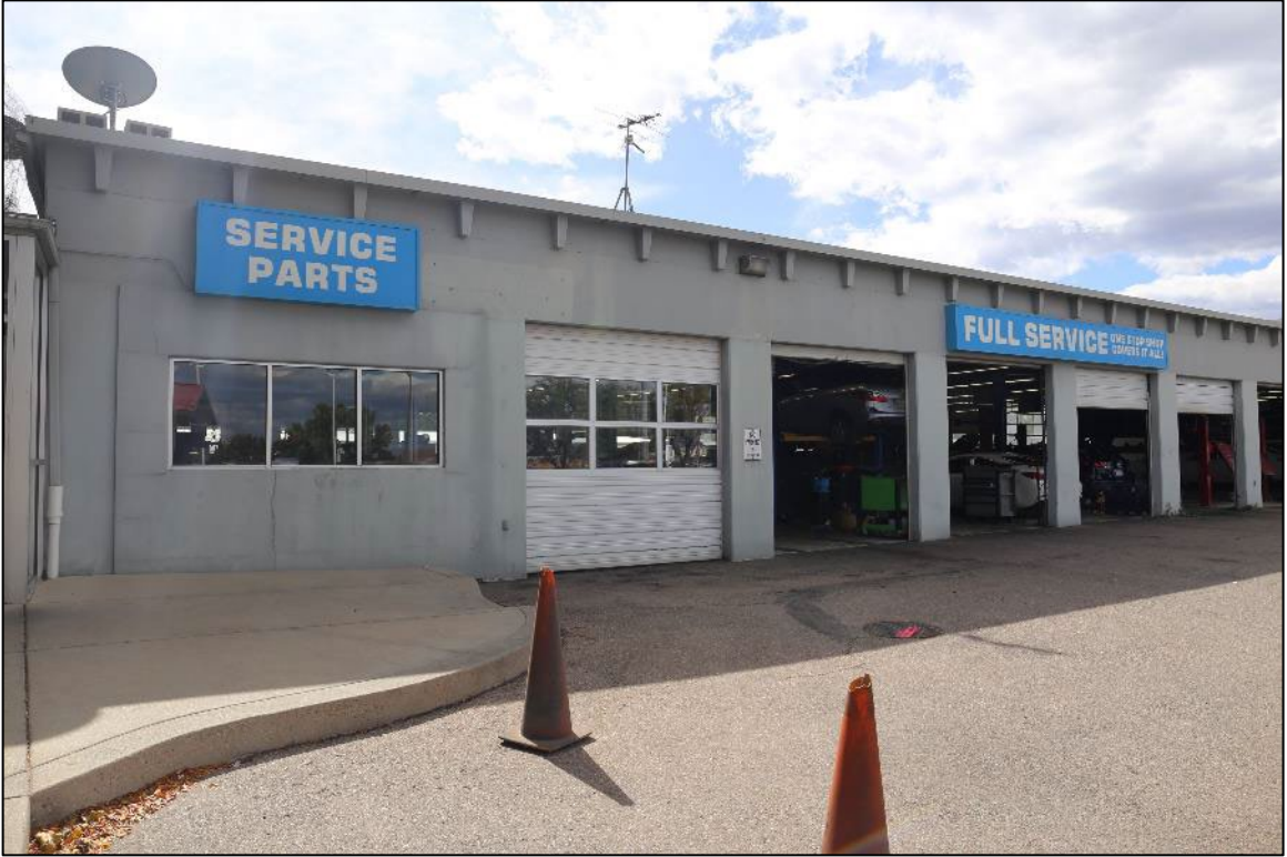
Figure 10: Feature 1, east half of north elevation, view south (Image #7221, R. Schields, 10/3/2023).
