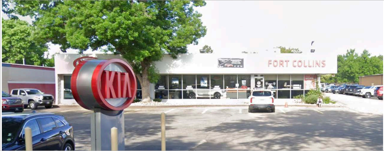
70. Kia dealership, 2849 South College Ave, built in 1972, not eligible for landmarking per the City of Fort Collins Historic Resources Planning Map. Image courtesy of BEE. 2024.
