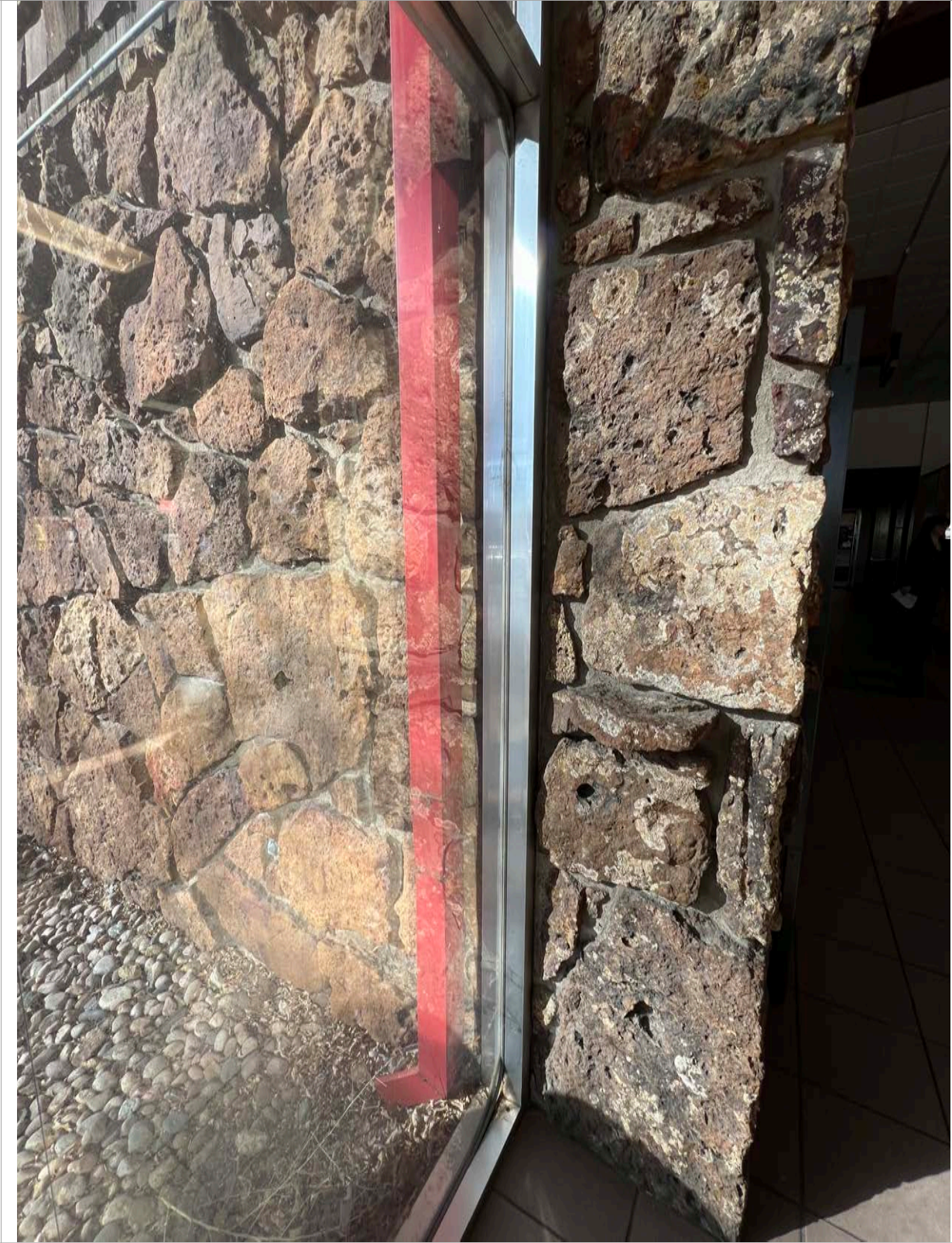
10. East Elevation - Image of connection of aluminum frame, single glaze window with stone veneer. Image courtesy of BEE. 2024.
