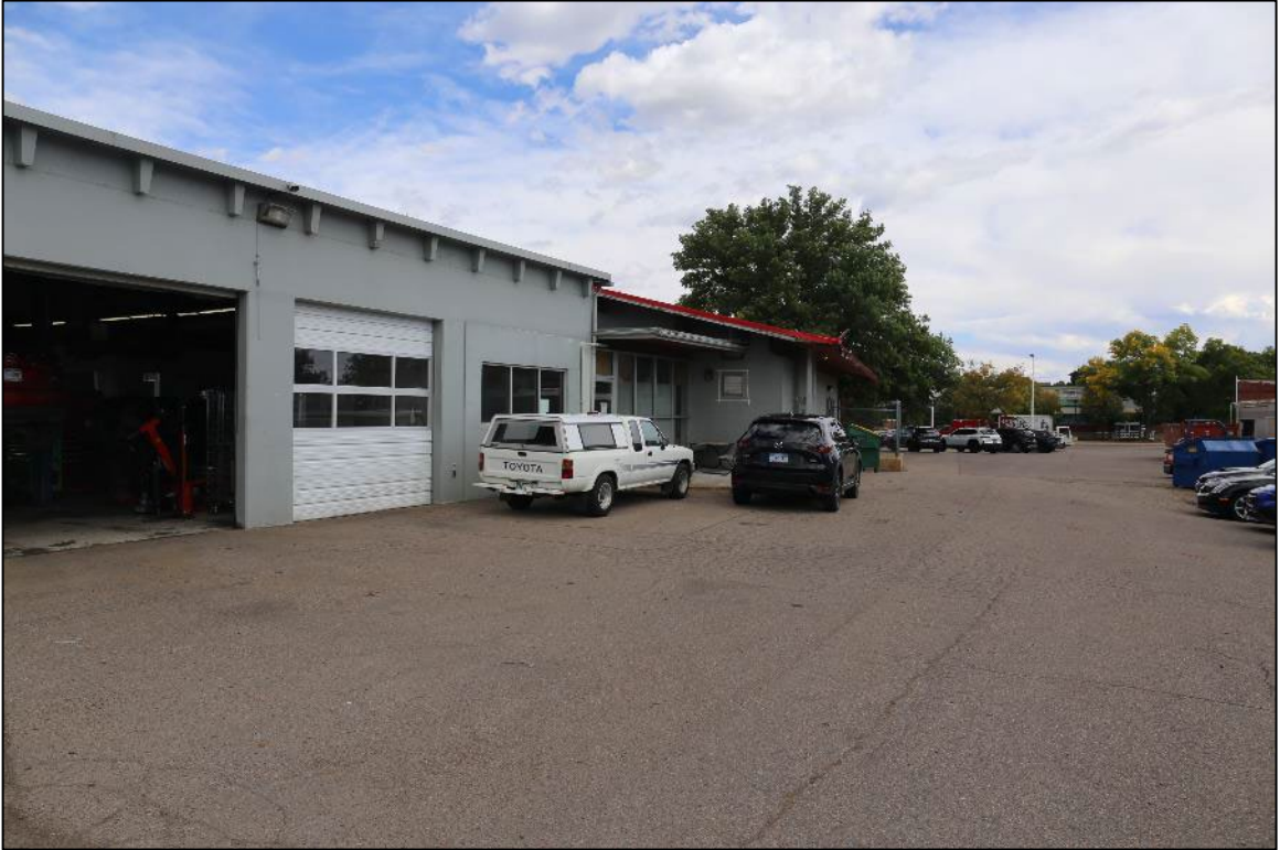
Figure 17: Feature 1, east end of south elevation. Note glass enclosed foyer between west and east portions of the building. (Image #7251, R. Shields, 10/3/2023).
