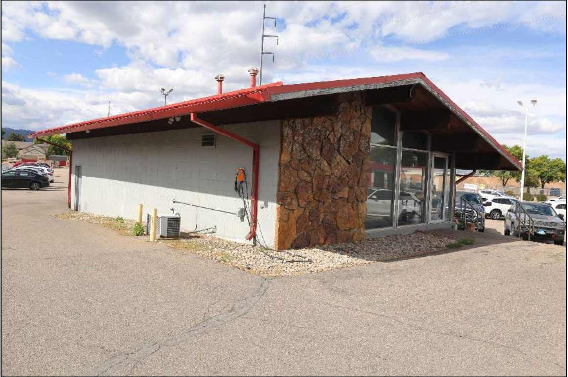
Figure 23: Feature 2, south-southeast and east-northeast elevations, view northwest (Image #7213, R. Schields, 10/3/2023).
