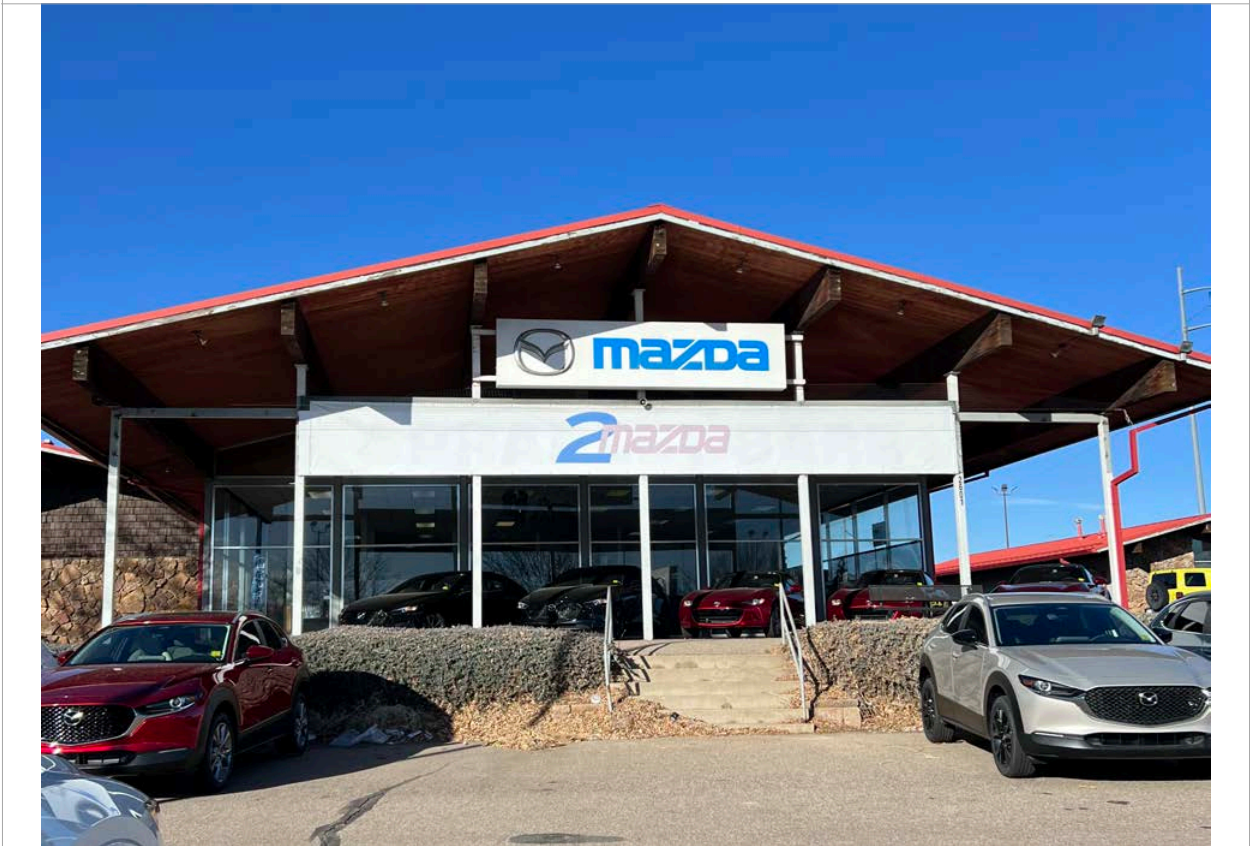
4. East Elevation - North end. Image courtesy of BEE. 2024
