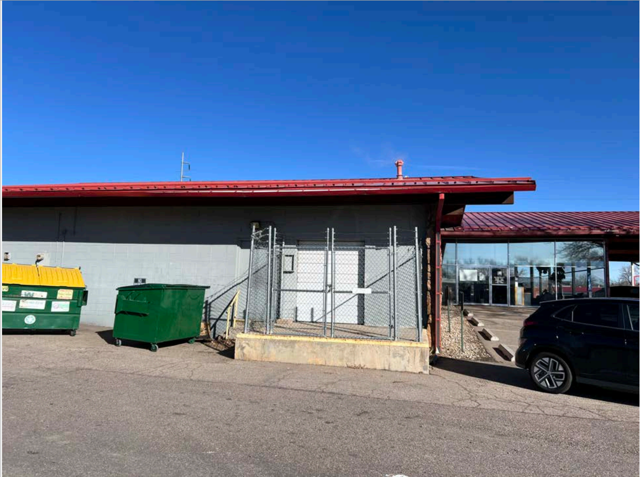
40. South Elevation - Showroom, SE corner of office portion. Showroom windows on photo right. Image courtesy of BEE. 2024.
