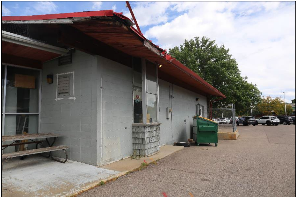
Figure 18: Feature 1, south-southeast elevation, view northeast. Note bump out, likely used as a drive through for part sales. (Image #7244, R. Shields, 10/3/2023).
