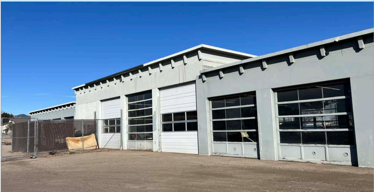
32. South Elevation - Service center, bays 7-15. Image courtesy of BEE. 2024.
