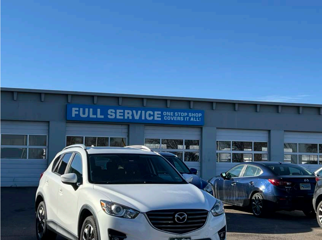
16. North Elevation - Service center, bays 3-6. Image courtesy of BEE. 2024.
