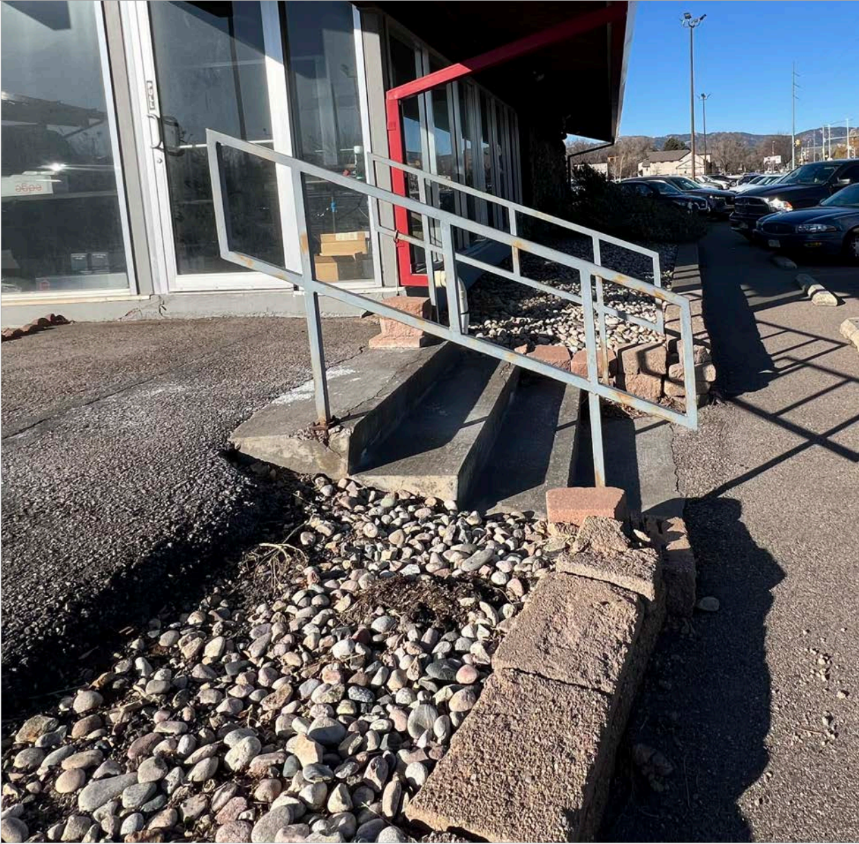
52. Site - Detail of stairs on north side of showroom. Image courtesy of BEE. 2024.
