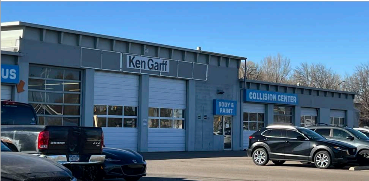
18. North Elevation - Service center, bays 9-11. Note the garage doors on bays 9 and 13 are original, all others have been replaced. Image courtesy of BEE. 2024.
