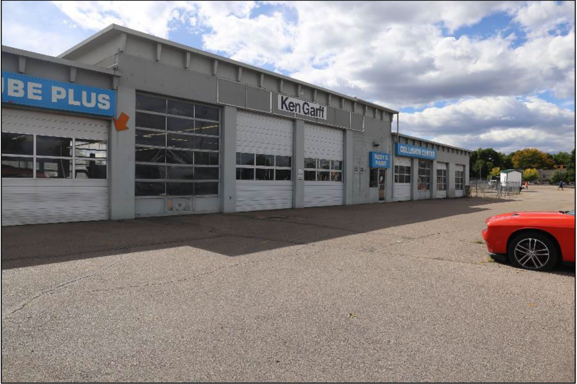
Figure 12: Feature 1, west half of north elevation, view southwest (Image #7224, R. Shields, 10/3/2023).
