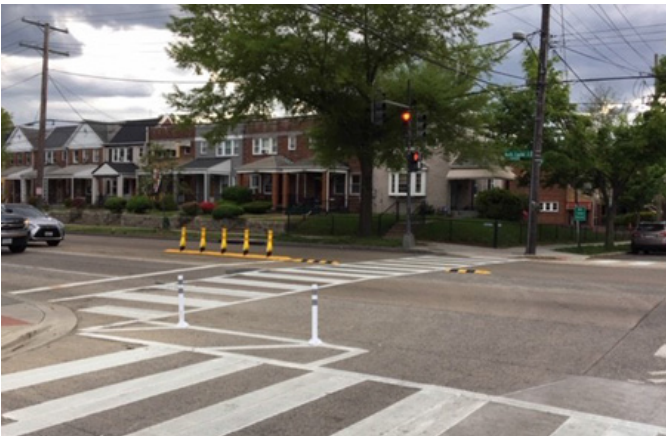
Figure 10: Flexible Delineators and Hardened Centerline to Control Turning Speed
