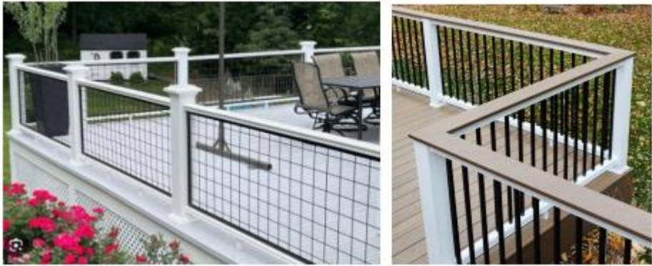
Railings: Type- Intermediate wooden newel post with cap and railing panel in between. Finish Material – Wood and metal Colors- white/black
