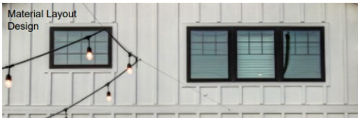
Exterior Siding: Board and Batten
