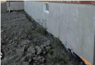
Foundation Wall: Exposed Concrete
