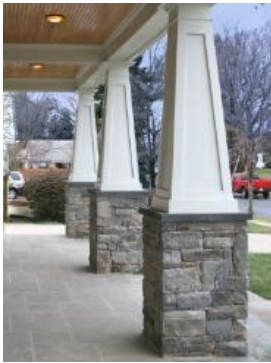
Columns: Stone Base Columns
