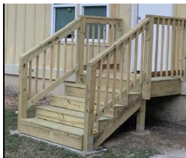
EXTERIOR STAIRS: WOOD
