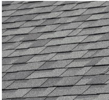
Roof: Fiberglass Shingles Roof
