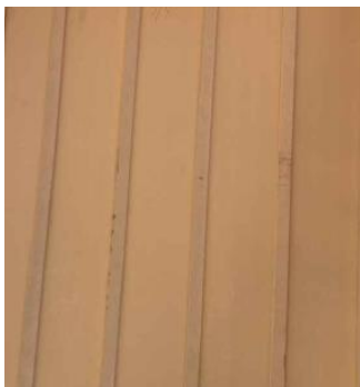
Exterior Siding: Board & Batton Siding
