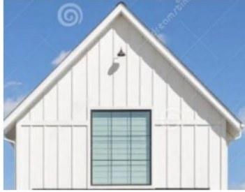
Exterior Siding: House Front will be cement based board & batten ( I.E. Hardie Siding)
