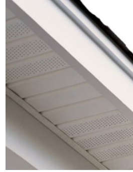
Soffit: Vinyl Soffit, Metal Wrap Fascia
