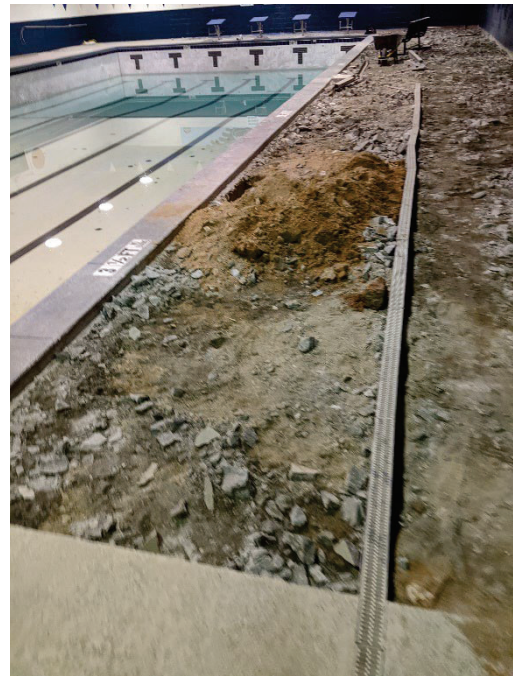
Photo 4 Review of slab removal
