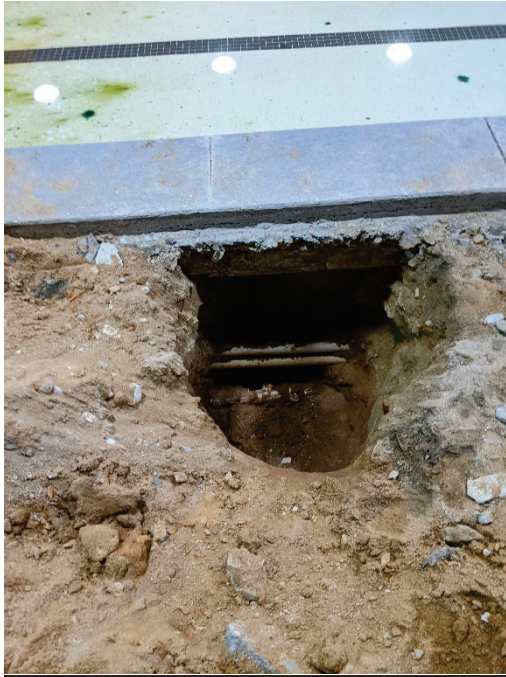
Photo 5 Review of excavation at leak
