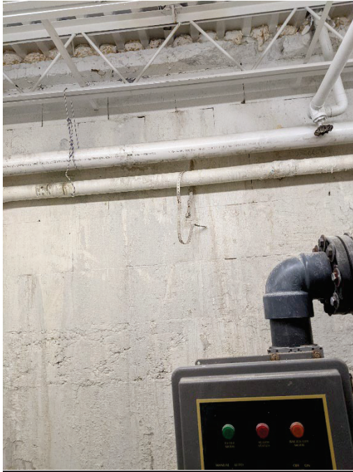
Photo 1 Southern Pool Wall/Equipment Room Wall
