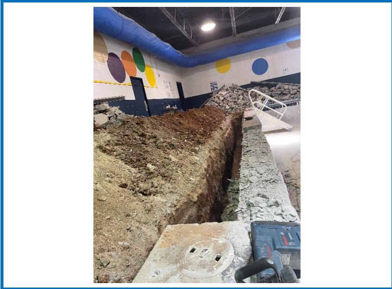
Photo 9: Excavated area N of pool. View from W. 5/2023
