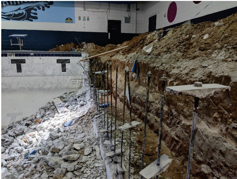
Photo 6 Review of Pool expansion excavation
