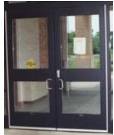
Front & Rear Doors: Metal Double Doors. Painted Metal: Color Black
