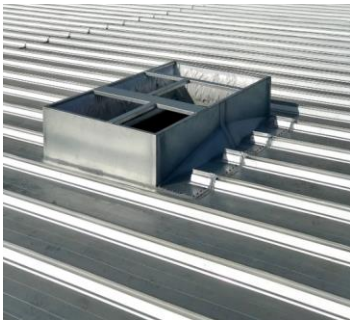
Roof: Mechanical Metal Roof.
