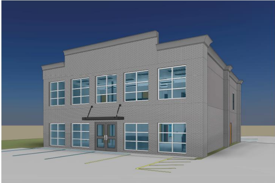
1 FRONT BUILDING VIEW
