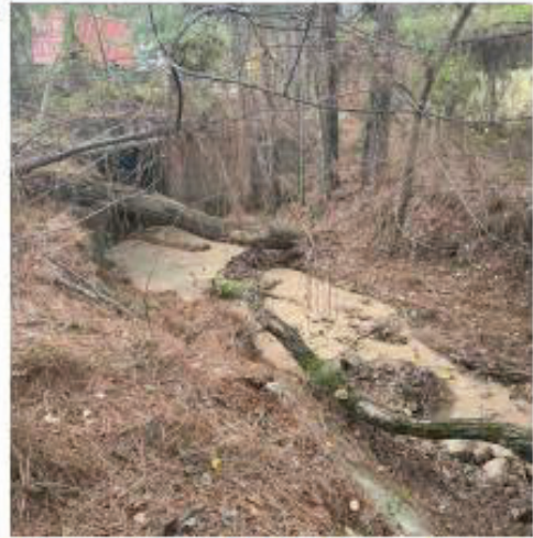
4 Ephemeral Channel 1 at Culvert Entrance near Moreland Ave
