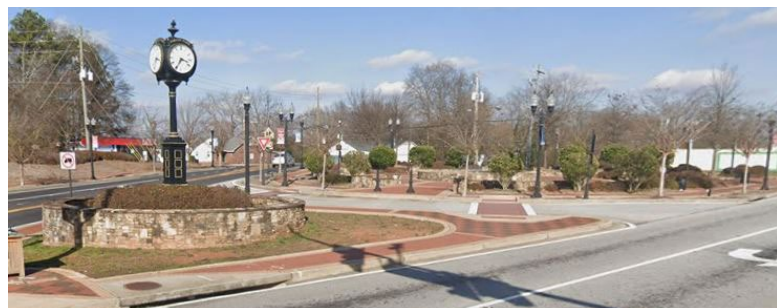
Roadway improvements along Main Street
