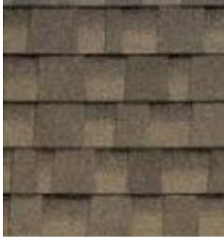
Roof Above Front Porch: Shaker Shingles
