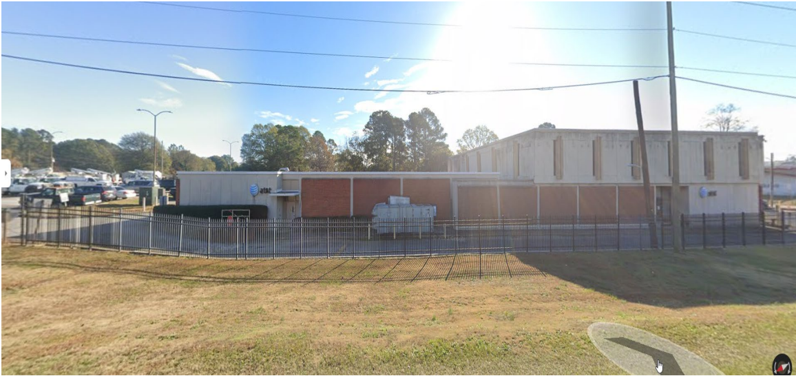
AT& T Telephone utility: GC (General Commercial)
