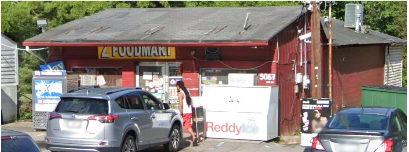
FRONT FAÇADE (MARCH 2023)
