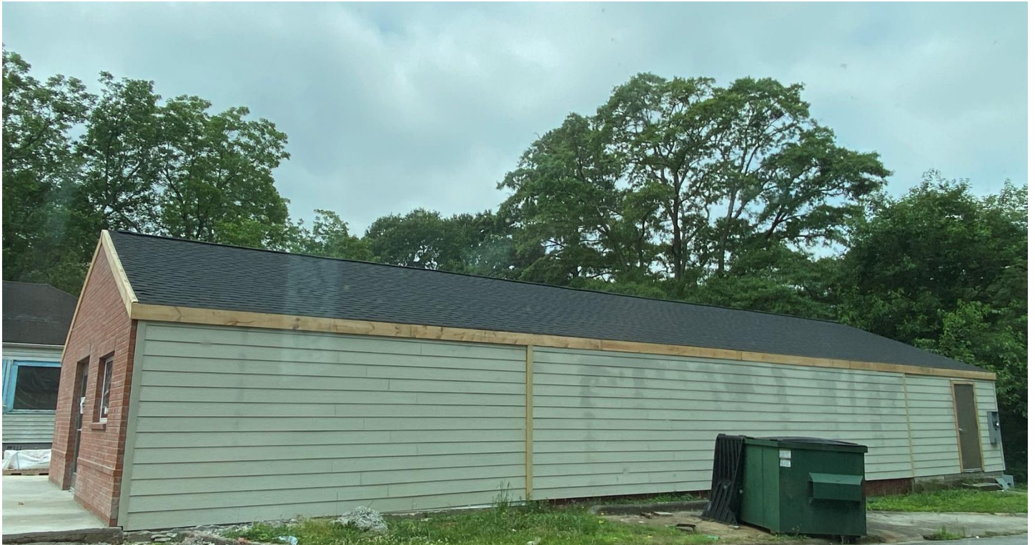
SIDE FAÇADE FACING BRIDGE AVE (JUNE 2023)
