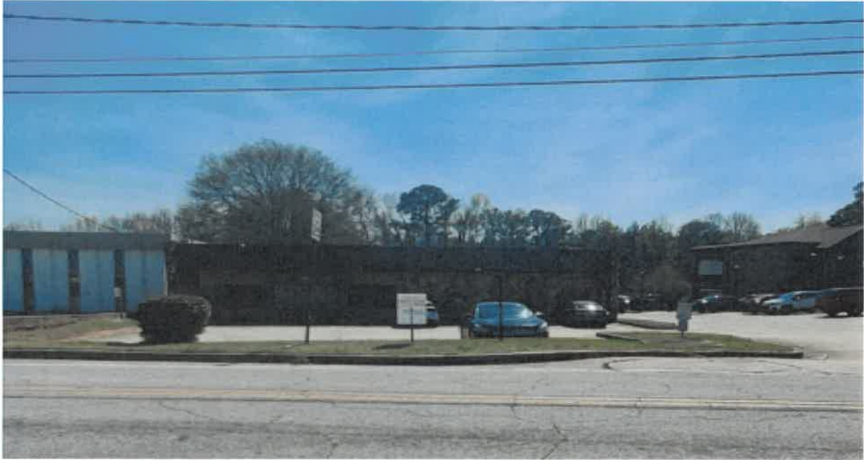
Vacant, Boarded Up Building
