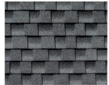
Roof: Asphalt Roof Shingles. GAF Timberline HDZ PEWTER GRAY
