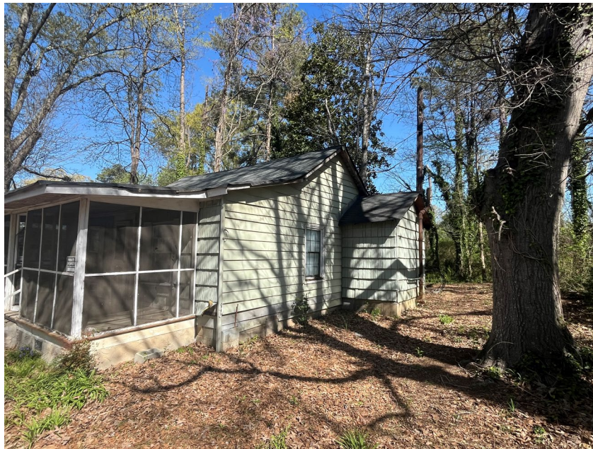
Side – East View
