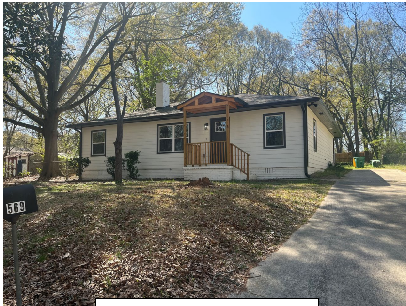
Side – East View
