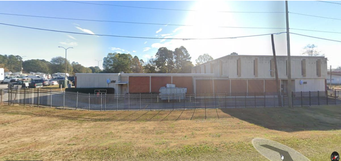
AT& T Telephone utility: GC (General Commercial)
