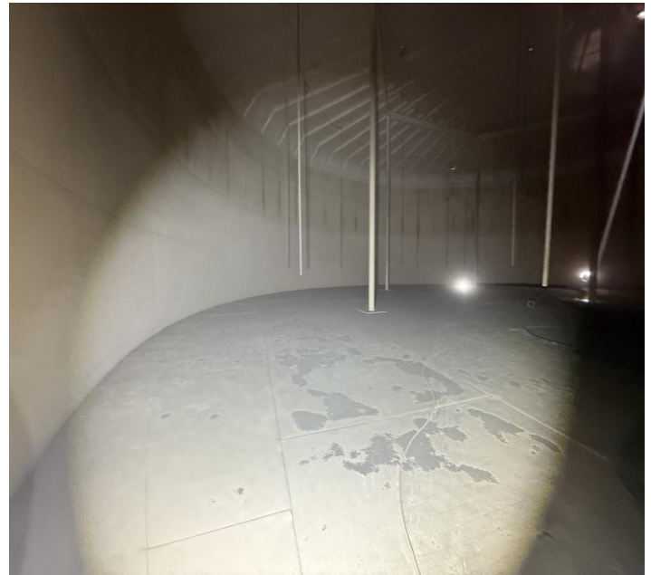
Interior floor of the Foothill Tank. Picture #2
