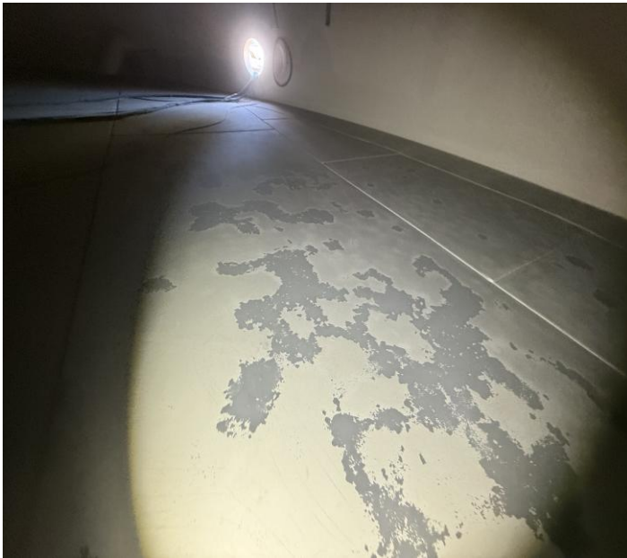
Additional photos of exposed substrate. Picture #1
