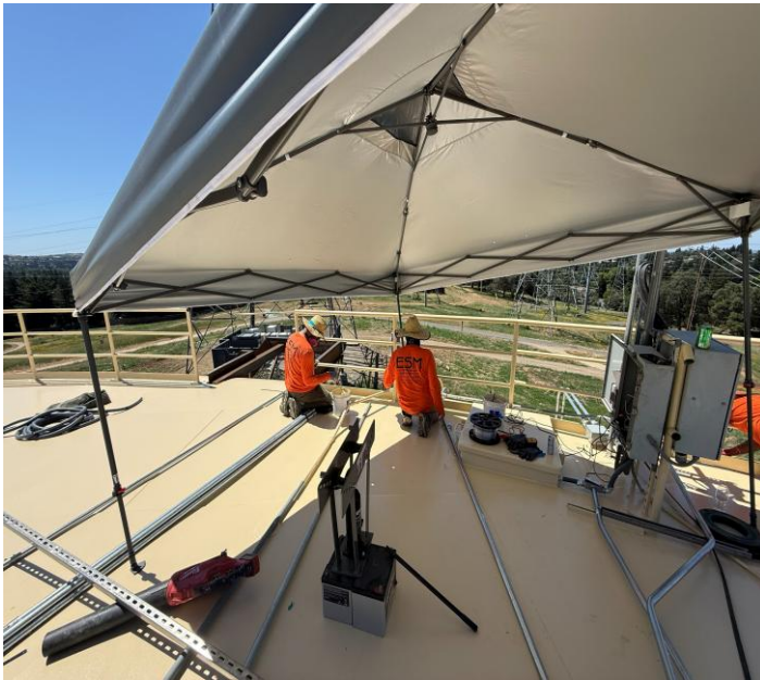
ESM crew members continuing 2 nd finish coat application. Picture #2
