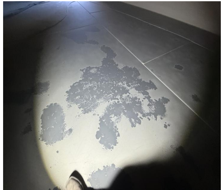
Additional photos of exposed substrate. Picture #2
