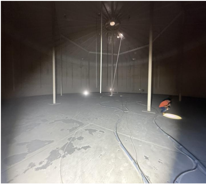
Interior floor of the Foothill Tank. Picture #1
