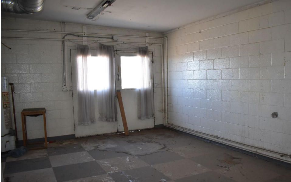
VIEW OF THE INTERIOR OF THE BUILDING
