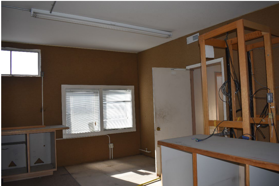
VIEW OF THE INTERIOR OF THE BUILDING
