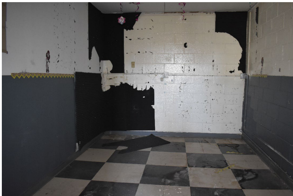
VIEW OF THE INTERIOR OF THE BUILDING
