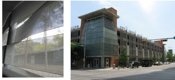
Figures 7-13 Illustrative Examples of Parking Garage Screening
